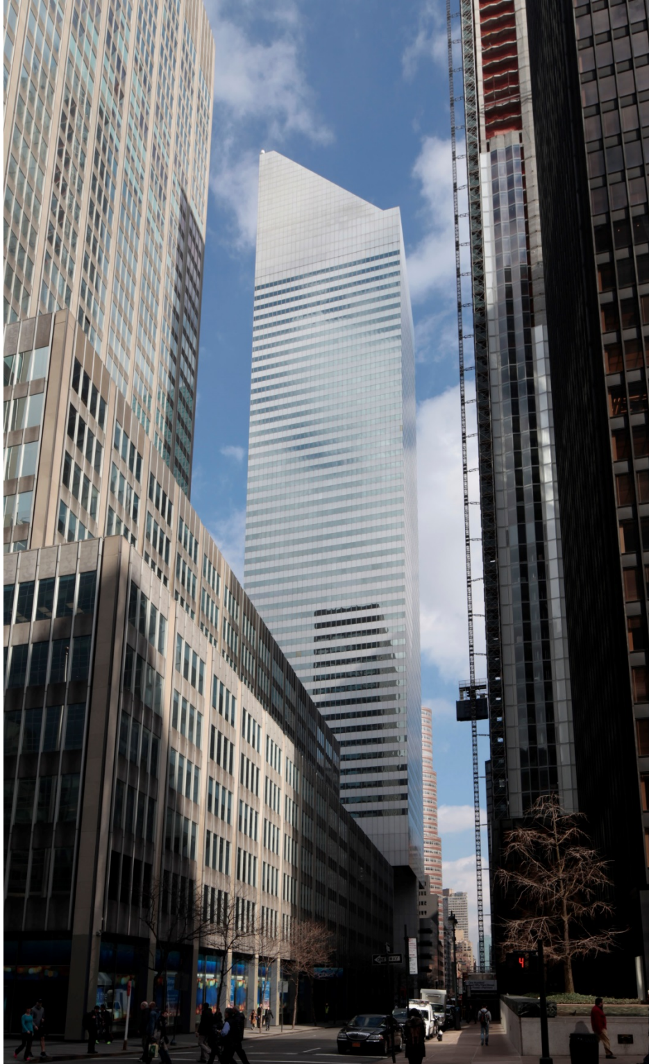
Citicorp Center (now 601 Lexington Avenue), including Saint Peter's Church Borough of Manhattan Tax Map Block 1308, Lot 7501 (1001, 1002, 1005) Office tower, west facade, viewed from Park Avenue and 53 rd Street Photo: Jenna Adams, 2016
