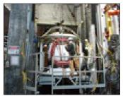
Now: Over 50 years later, DEP is doing extensive work on the same section of the Rondout-West Branch Tunnel. A special team of six divers was enlisted in 2008 to repair a valve 700 feet below the surface so that the tunnel can be dewatered and repaired. This image shows a member of
