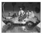
*I ben*: This image shows a 1957 inspection of the Rondout-West Branch portion of the Delaware Aqueduct. Board of Water Supply Engineers used a specially modified Jeep from the contractor to inspect a portion of the tunnel. The inspection report found the tunnel concrete lining to be
