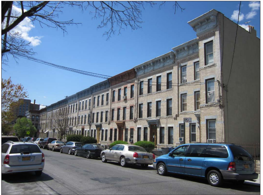
View southwest on Stanhope Street 8
