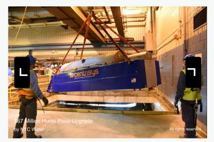
New Dewatering Centrifuges to Consume 60 Percent less Electricity, Approximately Equivalent to the Annual Electricity Use of 440 Homes; Avoiding Release of 826 Metric Tons of **Greenhouse Gases Annually**
