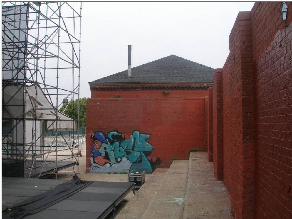
McCarren Play Center filter house: bleacher area and south elevation of northern filter house building, looking north. Stage and pool are to the left. Photo: Kathryn Horak, 2007
