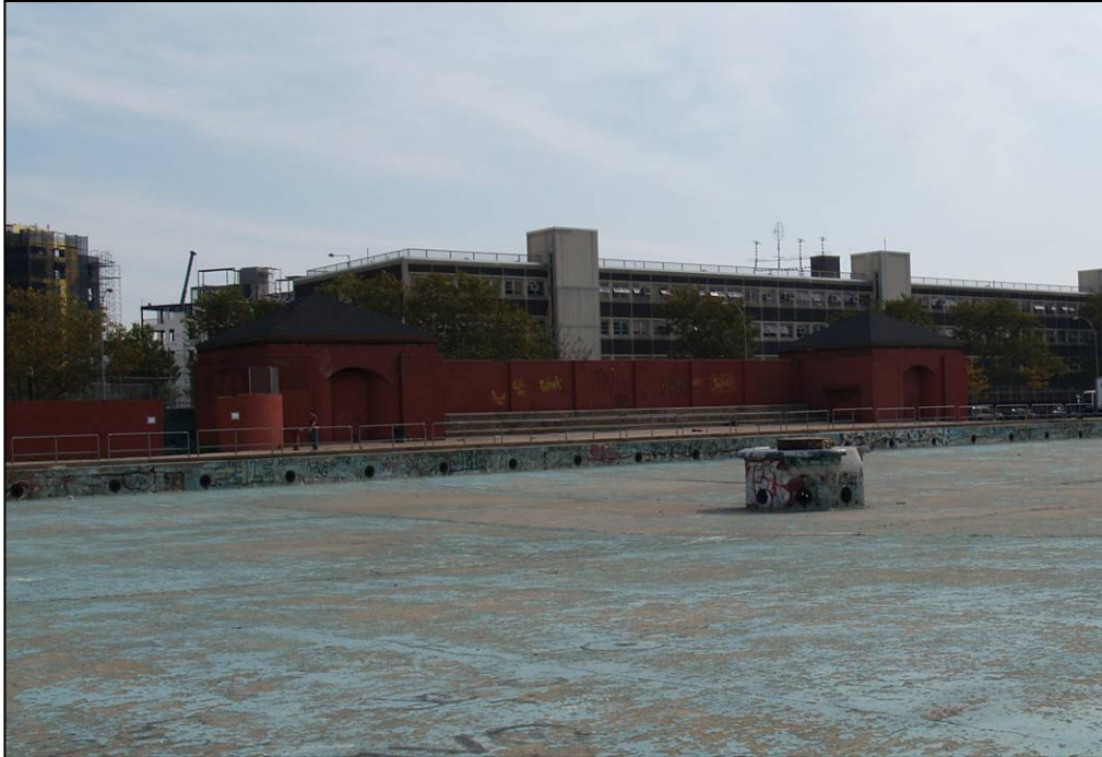
McCarren Play Center filter house: view looking southeast. Photo: Zerina Philip, NYC Parks Dept., 2006
