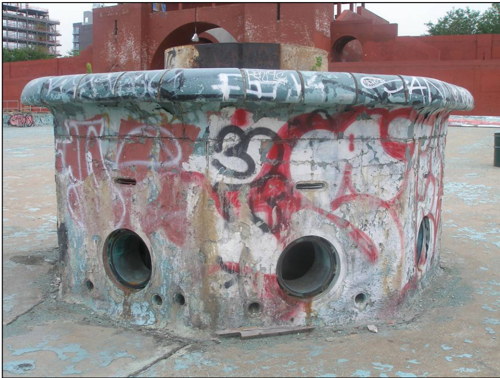
McCarren Play Center: pool, northern filter island. Looking southwest. Photo: Kathryn Horak, 2007
