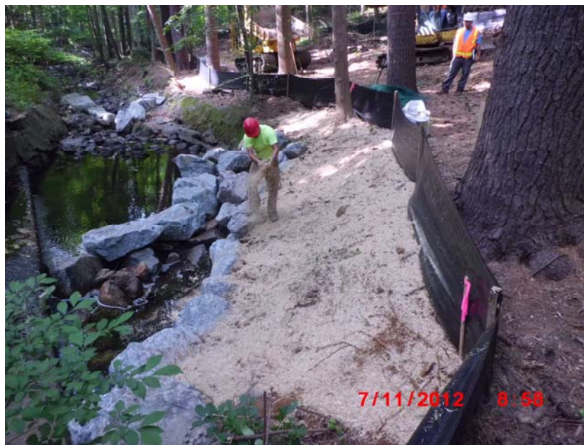
Seeding and mulching at Whippoorwill
