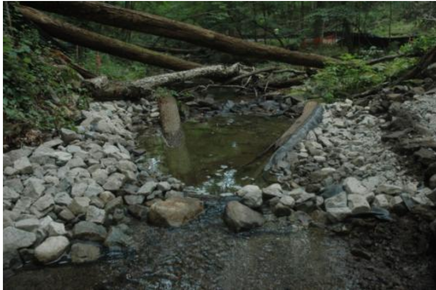
Log vane structure at Whippoorwill
