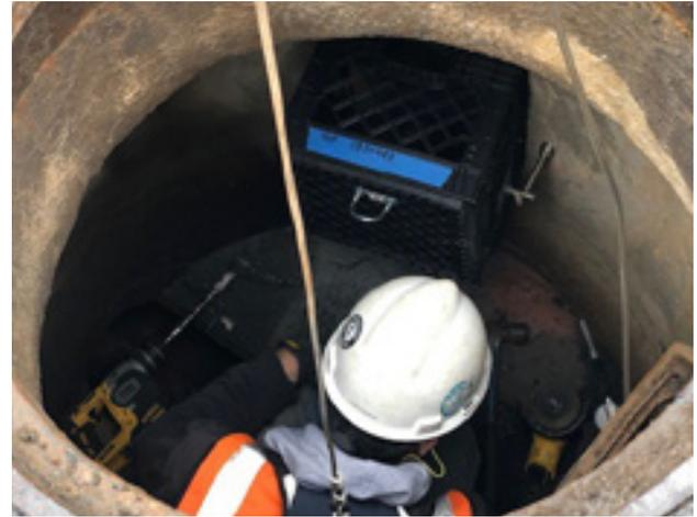
Loading Rate Study - Monitoring equipment installation
