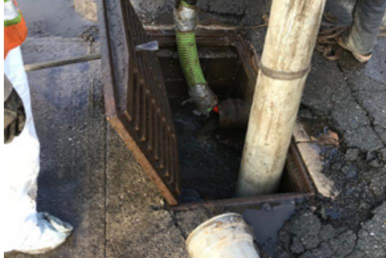
NYPD cleaning stormwater assets and installing filter fabric to prevent catch basin sediment accumulation.
