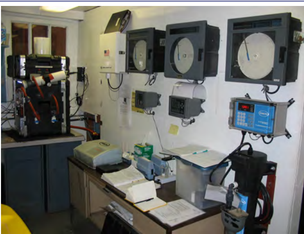
Figure 1.6 Continuously recording equipment used to monitor water quality in the aqueducts.
