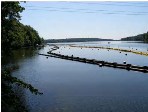
Figure 3.18 Turbidity curtain in Ken-sico Reservoir at the Catskill Upper Effluent Chamber (UEC) diverts stormwater away from the intake.
