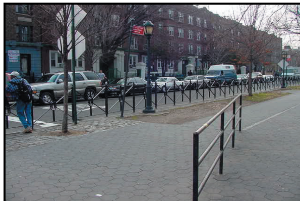
Pedestrian barriers along service road island prevent individuals from crossing service road midblock
