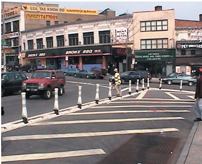
Flexible delineators and markings provide for increased pedestrian and vehicular safety
