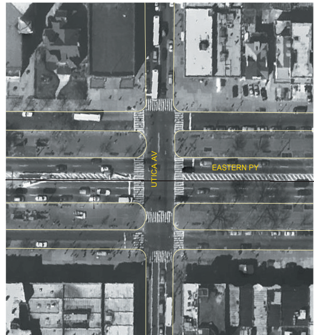
Aerial view of reconfigured intersection
