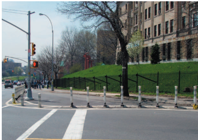
Reconfigured intersection and the use of bollards provides refuge and space for pedestrians.
