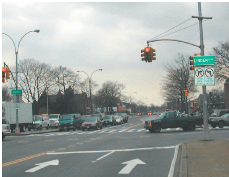
New markings, turning lanes and signage were installed to improve safety
