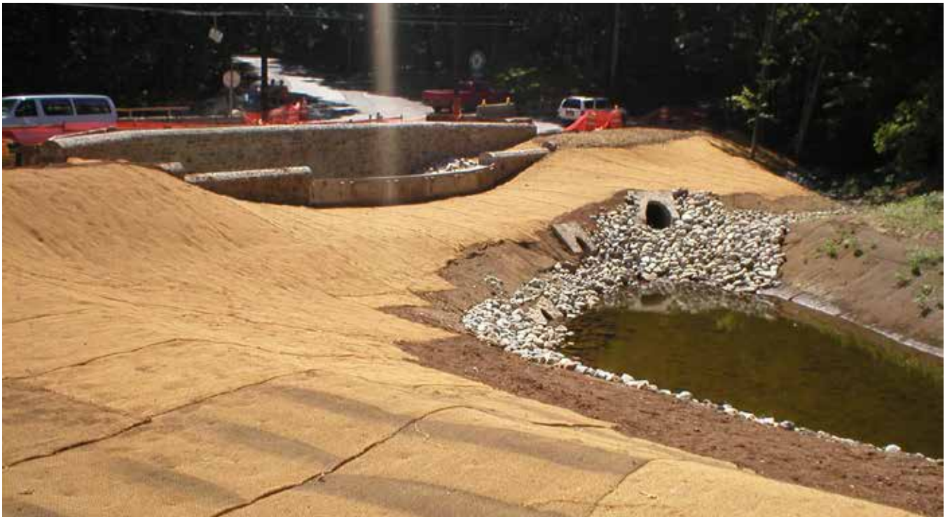
Erosion and sediment control measures in place during construction of a BMP in the Staten Island Bluebelt, NY
