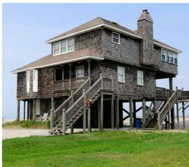
Houses meeting freeboard requirements in coastal areas by raising living spaces to the required height above the 100-year flood elevation
