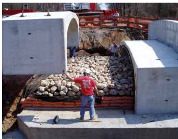
Rough bottom culverts were used to maintain fish passage
