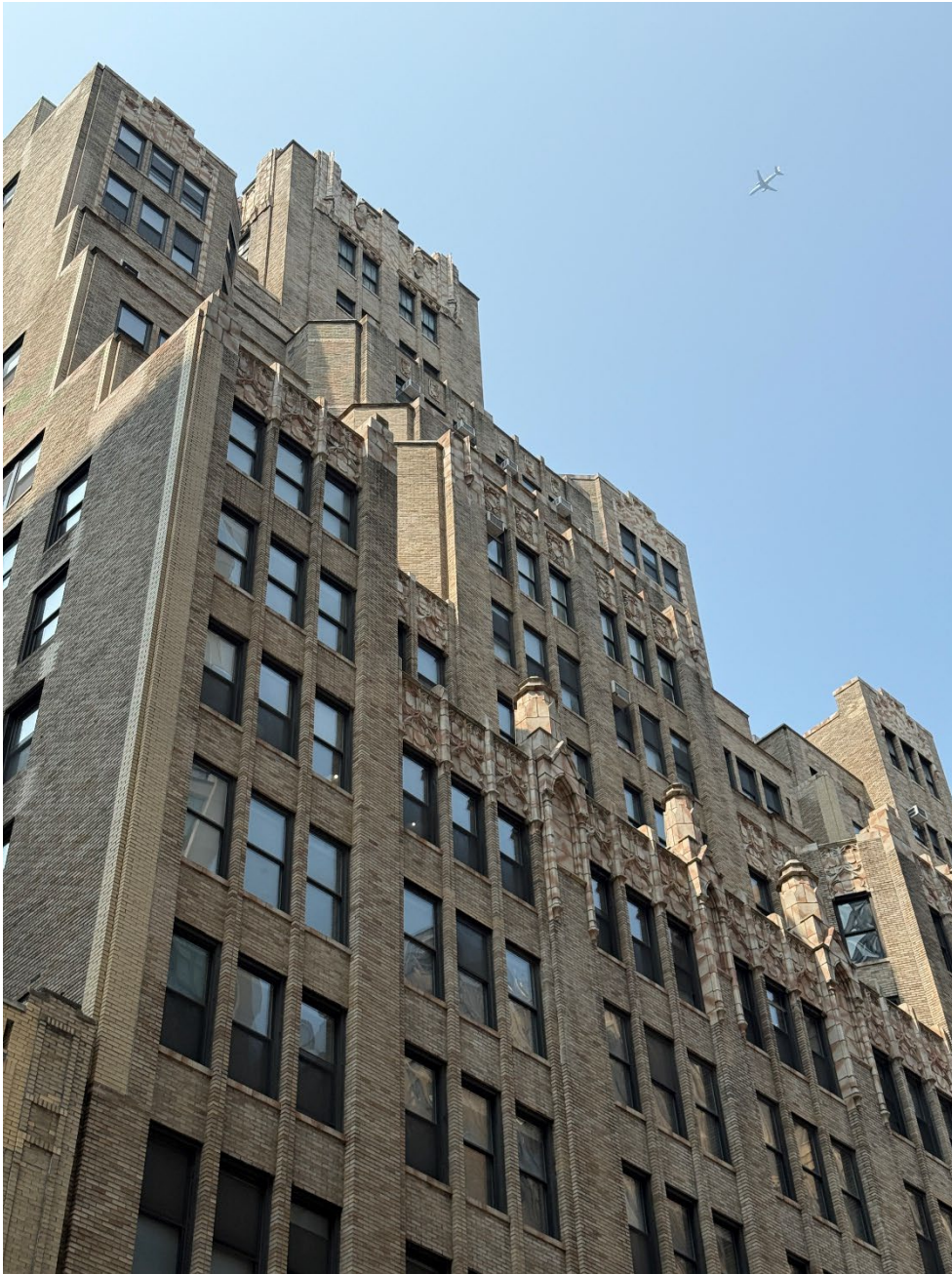
29th Street Towers, 214-226 West 29th Street
