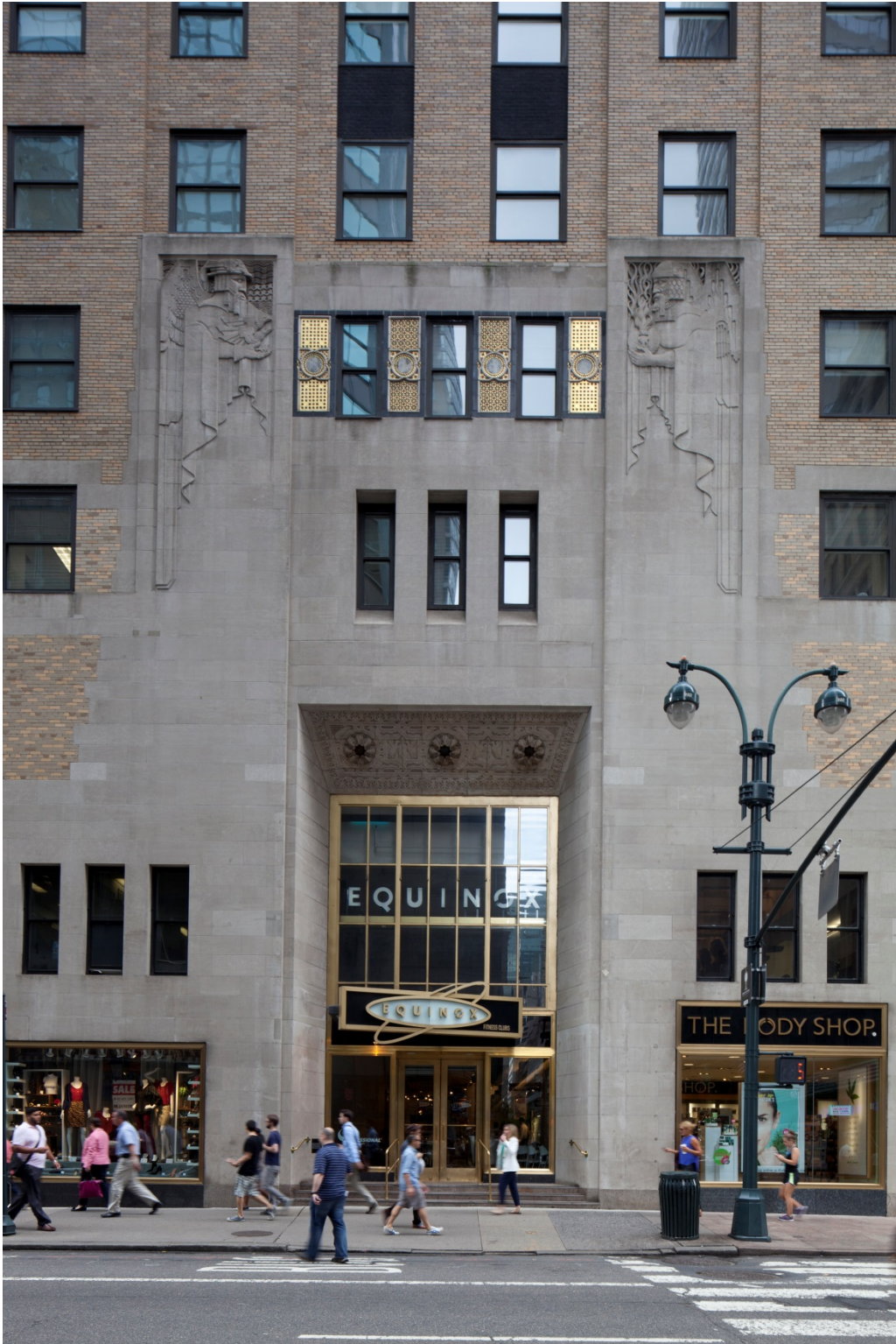
The Graybar Building North portal, 2013 Photo: Sarah Moses, 2016
