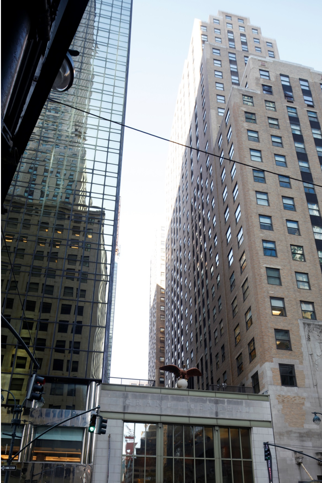
The Graybar Building South facade Photo: Sarah Moses, 2016
