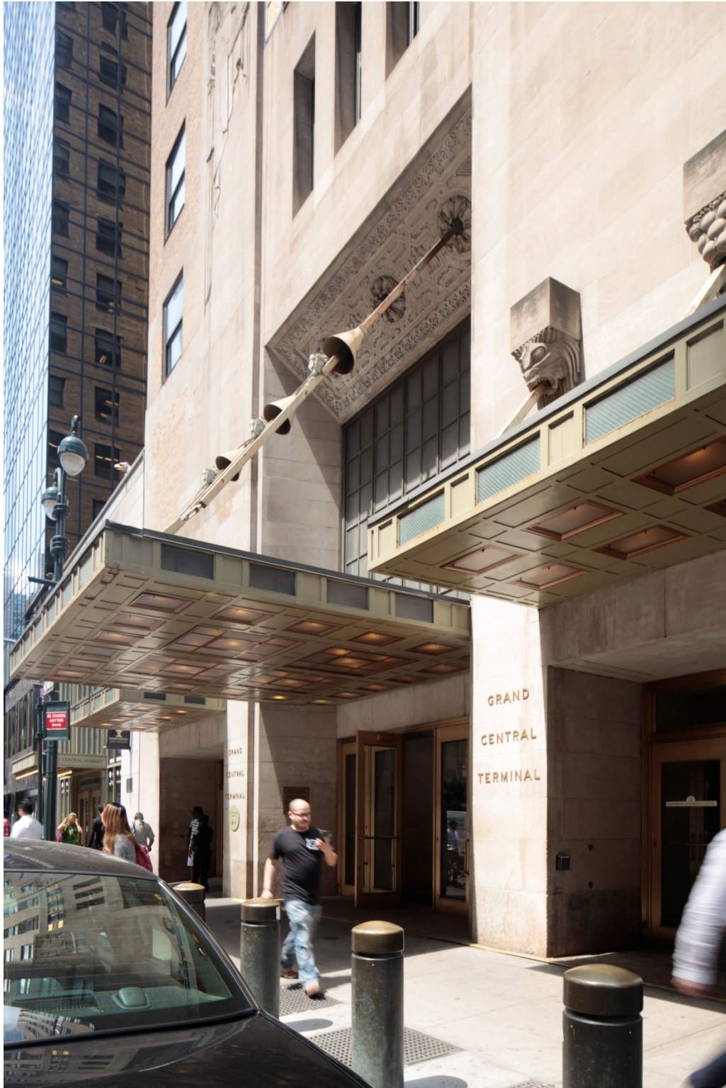
The Graybar Building South portal entrance with rat sculptures Photo: Sarah Moses, 2016
