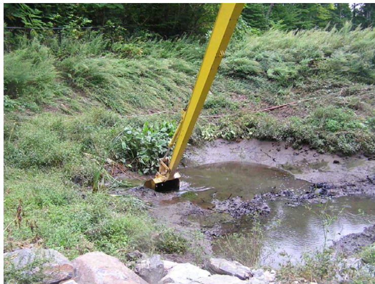
Figure 4.30 Photo of accumulated sediment being removed.
