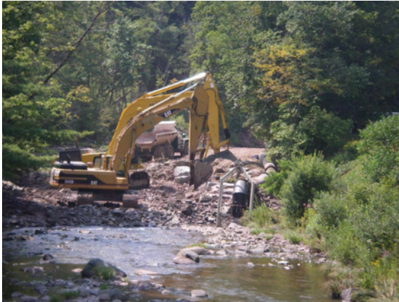
Figure 4.17b Long Road during restoration.
