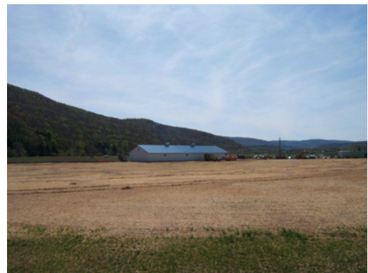
Figure 3.2. Hamden leach field and sand filter building.
