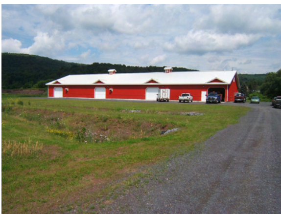
Figure 3.1. Bloomville sand filter building.
