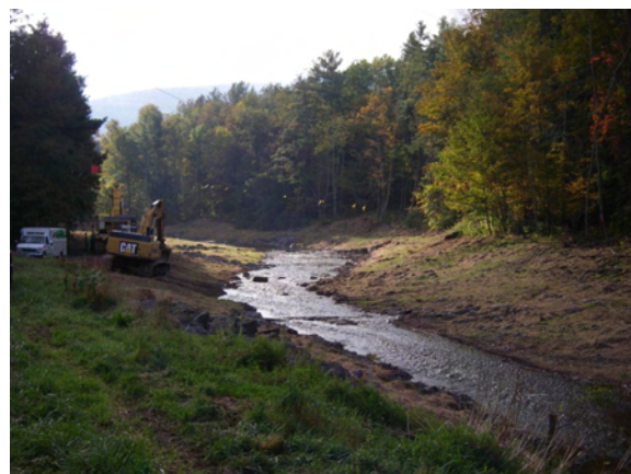
Figure 4.17c Long Road after restoration.
