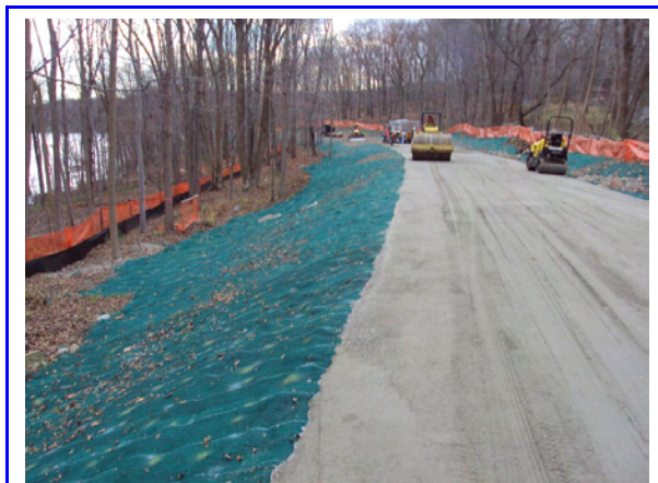
Figure 4.27 Completed erosion protection on slope.
