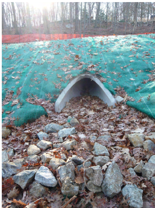
Figure 4.28 Completed drainage culvert with stone outfall protection.
