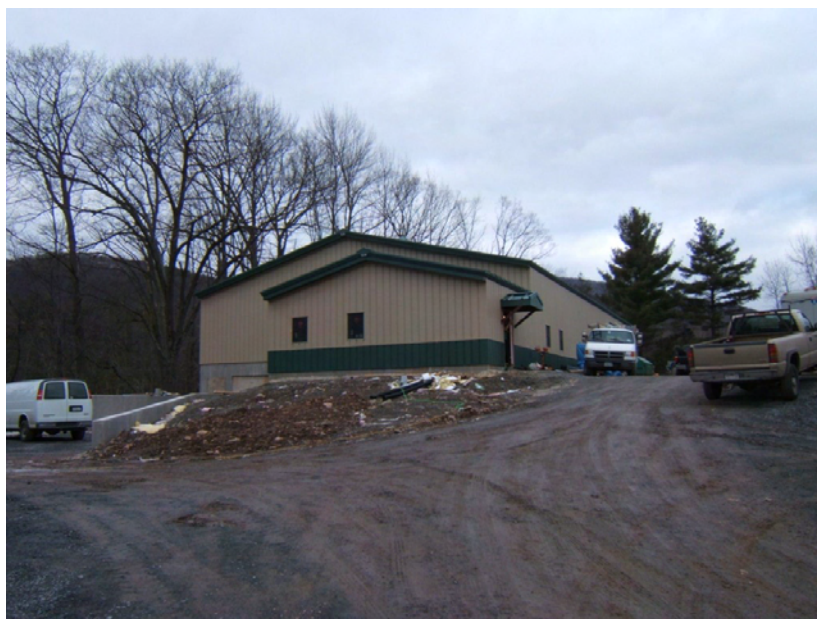
Figure 3.3. The Boiceville wastewater treatment plant.
