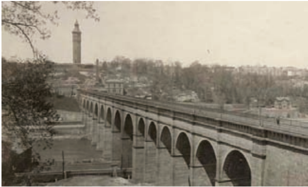
Old Croton Aqueduct
