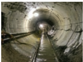
City Water Tunnel No. 3
