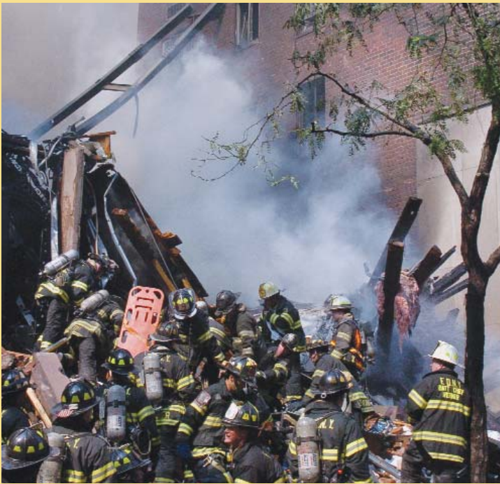
Manhattan Box 66-0947, 34 East 62nd Street/Madison Avenue, July 10, 2006. photo by FF Michael Gomez
