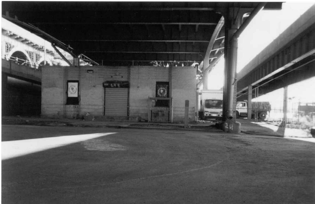
Figure 21.7-2 : Police precinct building located beneath Henry Hudson Parkway, on 135th Street.
