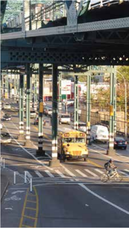
Pedestrian injuries declined 22% on New York City streets with protected bicycle lanes, like this one on Westchester Avenue.
