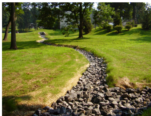
Figure 5.5 Stormwater swale repair.
