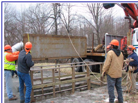
Figure 3.1 Stop Shutter Installation in the Catskill Aqueduct at Moodna, NY (J. Helmuth).
