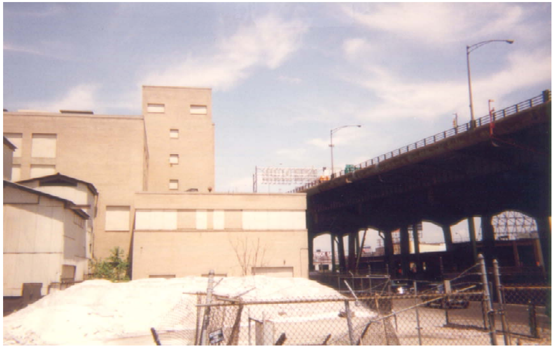
Figure 7.7-3 : View of the southern most portion of the site (salt storage area). (Photo 2000)
