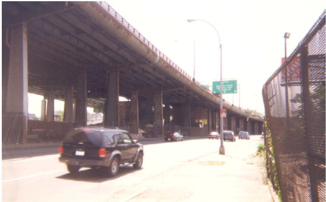
Figure 7.7-4 : View southward along Hamilton Avenue (and beneath the elevated Gowanus Expressway), adjacent to the site. (Photo 2000)
