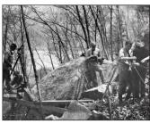
*hen*: A Board of Water Supply survey team on Storm King Mountain located on the west side of the Hudson River and from where the Catskill Aqueduct would cross the Hudson River on its route to New York City, May 10, 1907. The surveying instruments measured angles and a steel tape was used to calculate distances.
