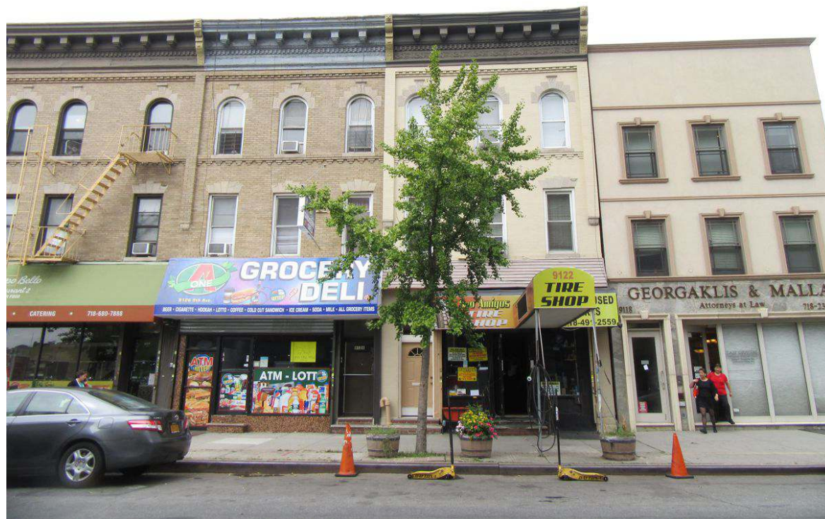
6. View of the Project Area facing northwest from 5th Avenue.
