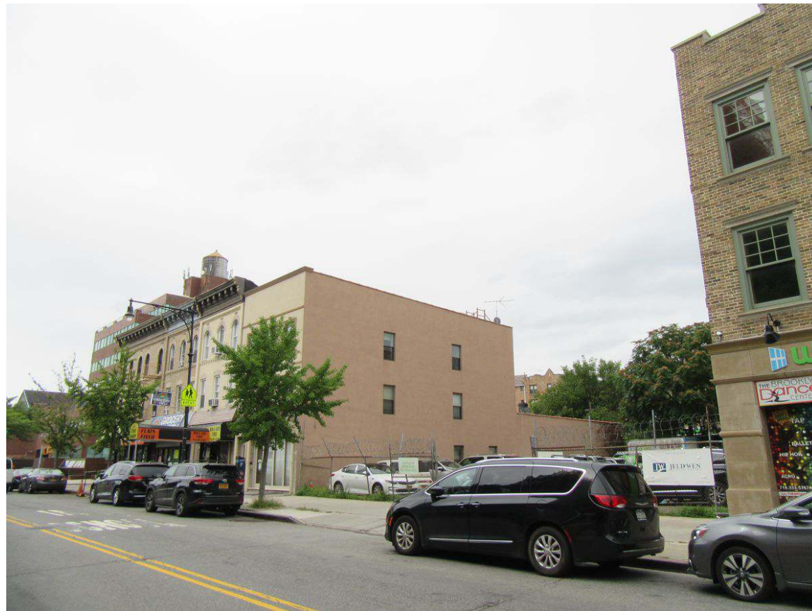
3. View of the Development Site facing west from 5th Avenue.
