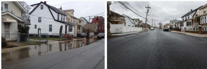
Sharon Chatman's street prior to construction (left) shows persistent ponding; after construction (right) the ponding is gone
