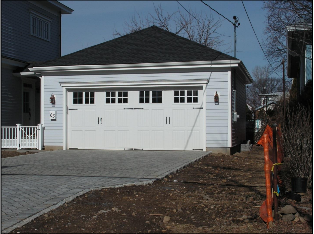
William H. Schofield House New Garage 65 Schofield Street (South East elevation) Photo: Theresa C. Noonan, 2016
