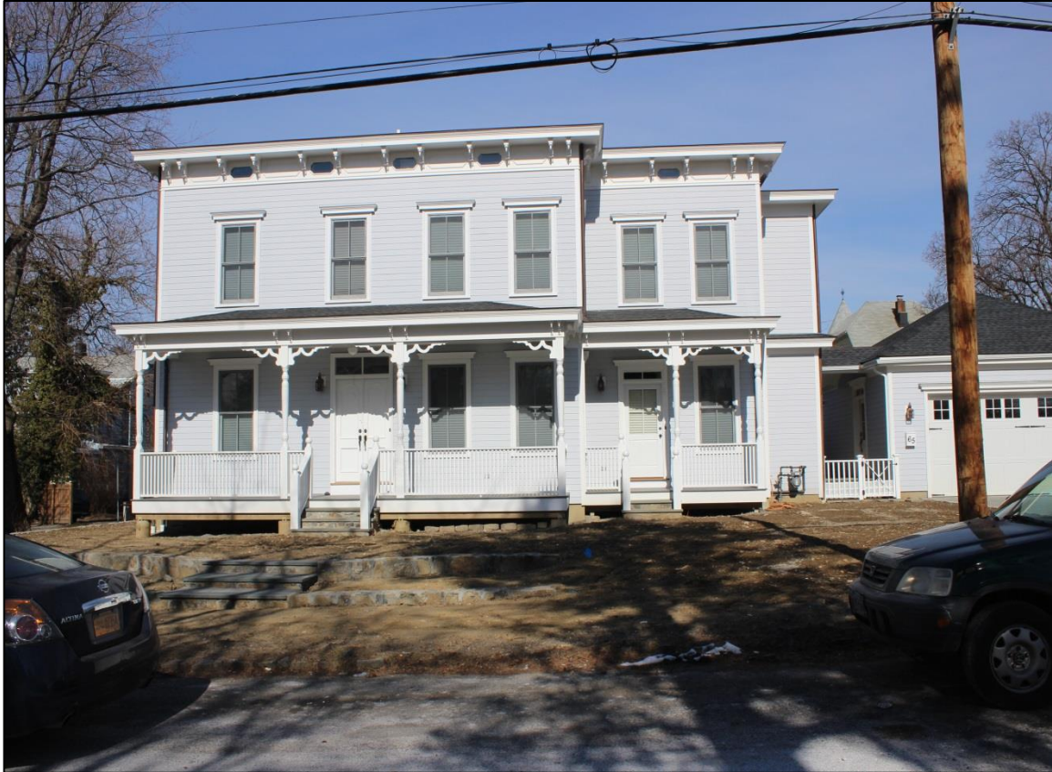
William H. Schofield House 65 Schofield Street (South elevation) Borough of the Bronx Tax Map Block 5628 Lot 146 Photo: Marianne Percival, 2016
