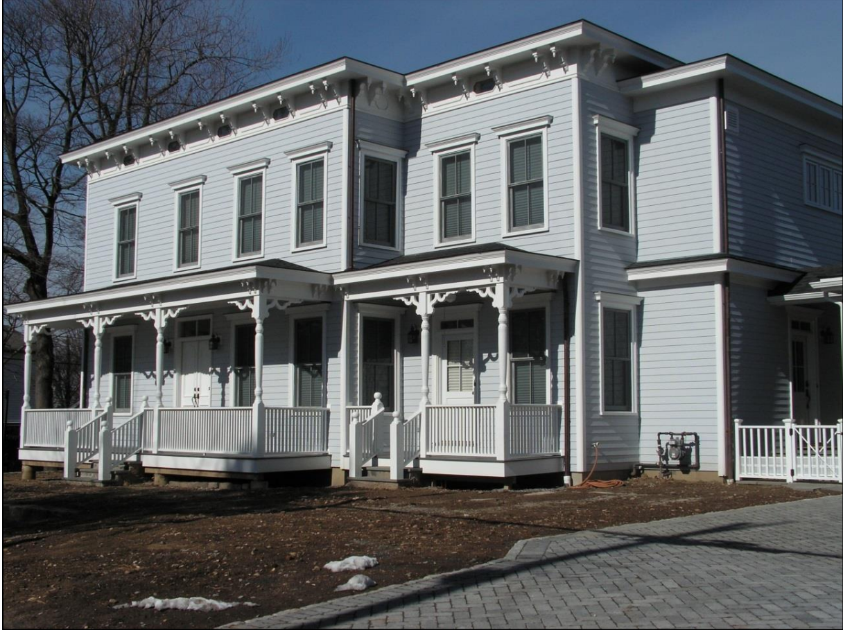
William H. Schofield House 65 Schofield Street (Addition) Photo: Theresa C. Noonan, 2016
