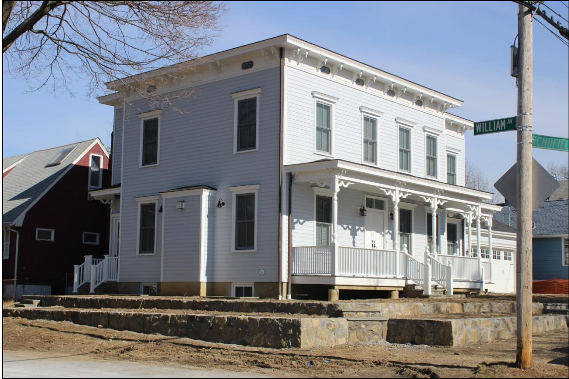
William H. Schofield House 65 Schofield Street (West elevation) Photo: Theresa C. Noonan, 2016
