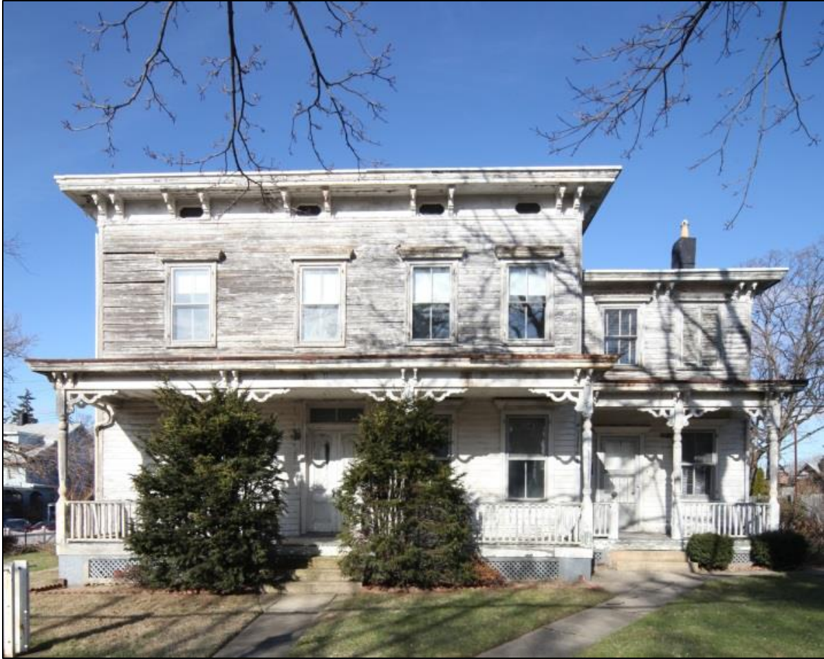
William H. Schofield House 65 Schofield Street (South elevation) Photo: Theresa C. Noonan, 2010
