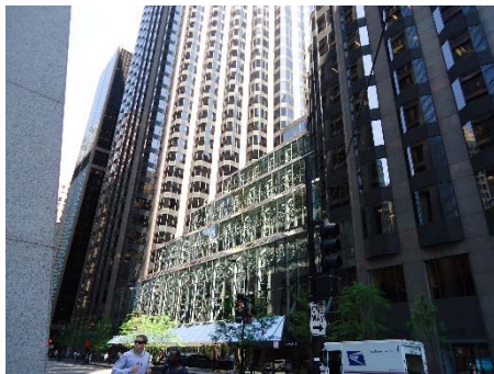
Figure 3: Terraced Facade in Toronto
