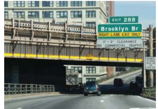
DOT improved bridge fascia over the BQE to reduce bridge strikes
