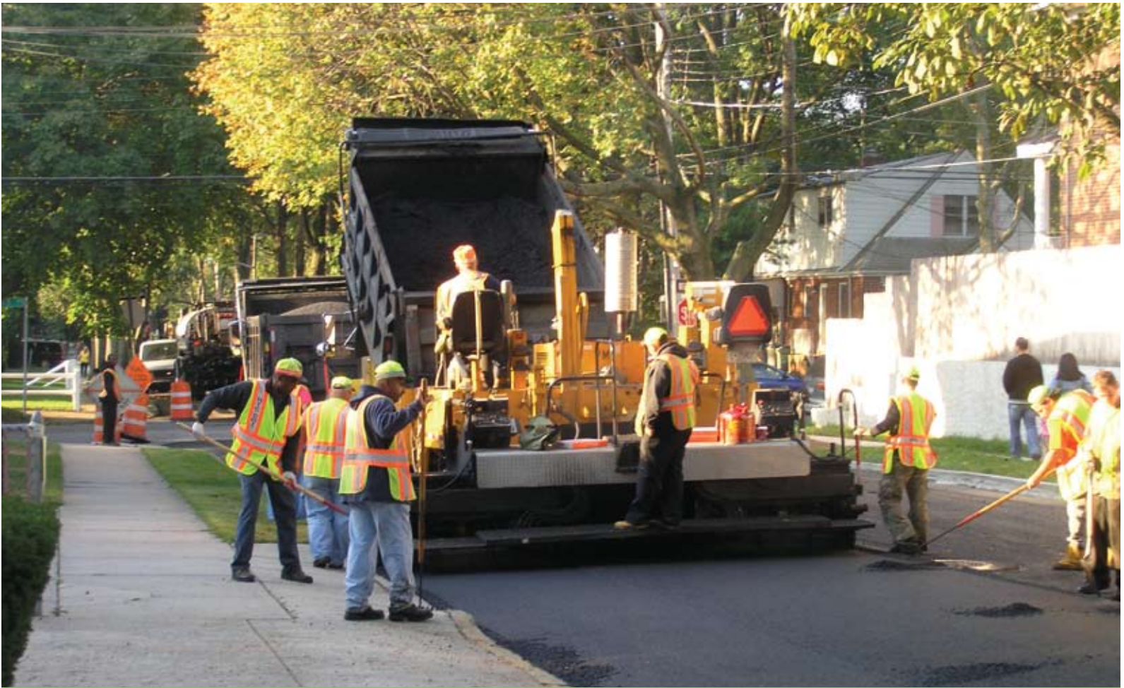
Warm mix asphalt being laid in Queens
