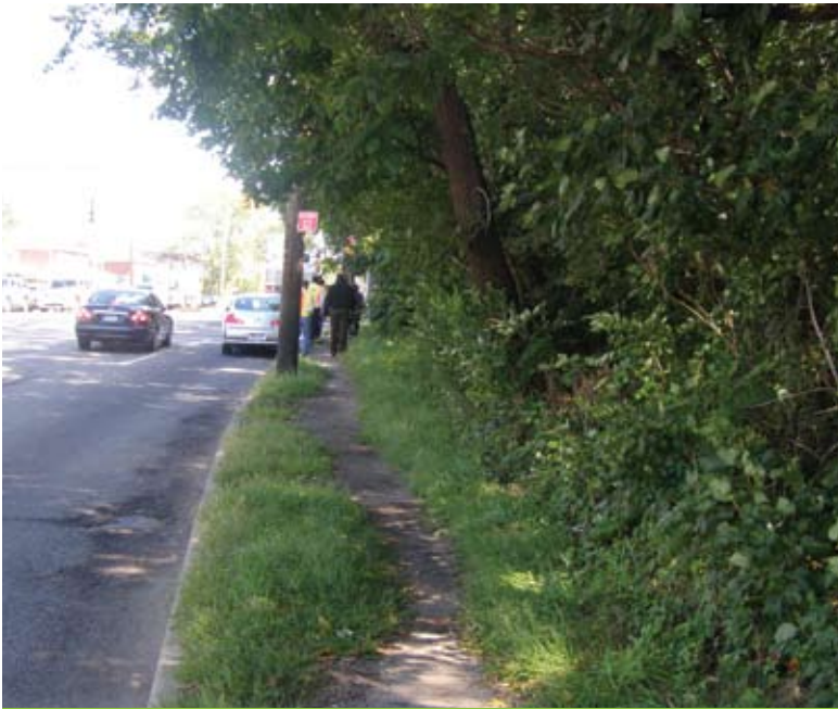
Before: Hylan Boulevard – No sidewalk
