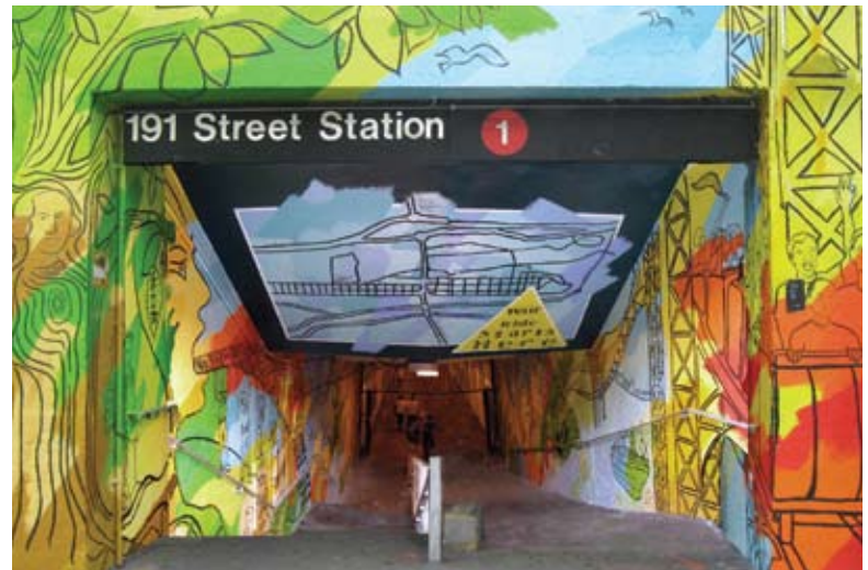
DOT's Urban Art program partners with community groups to create a mural at a newly refurbished pedestrian subway tunnel at 190th Street in Washington Heights
