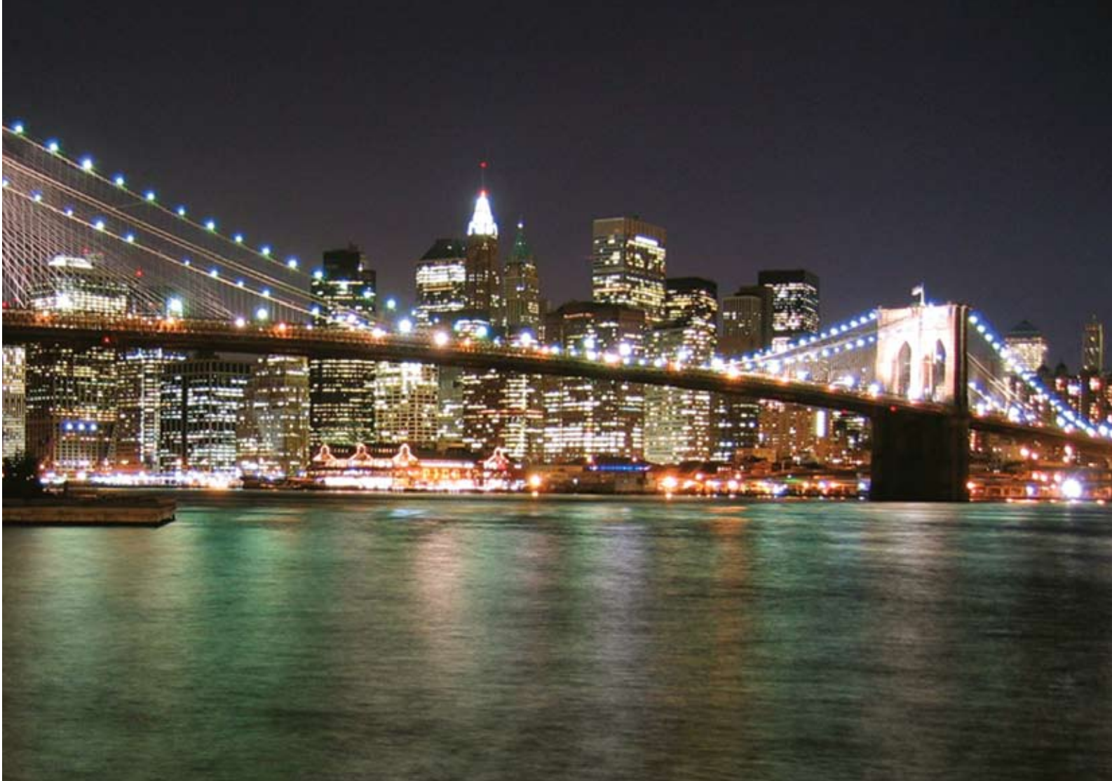
DOT will replace the necklace lights on all four East River bridges with energy efficient LED lights
