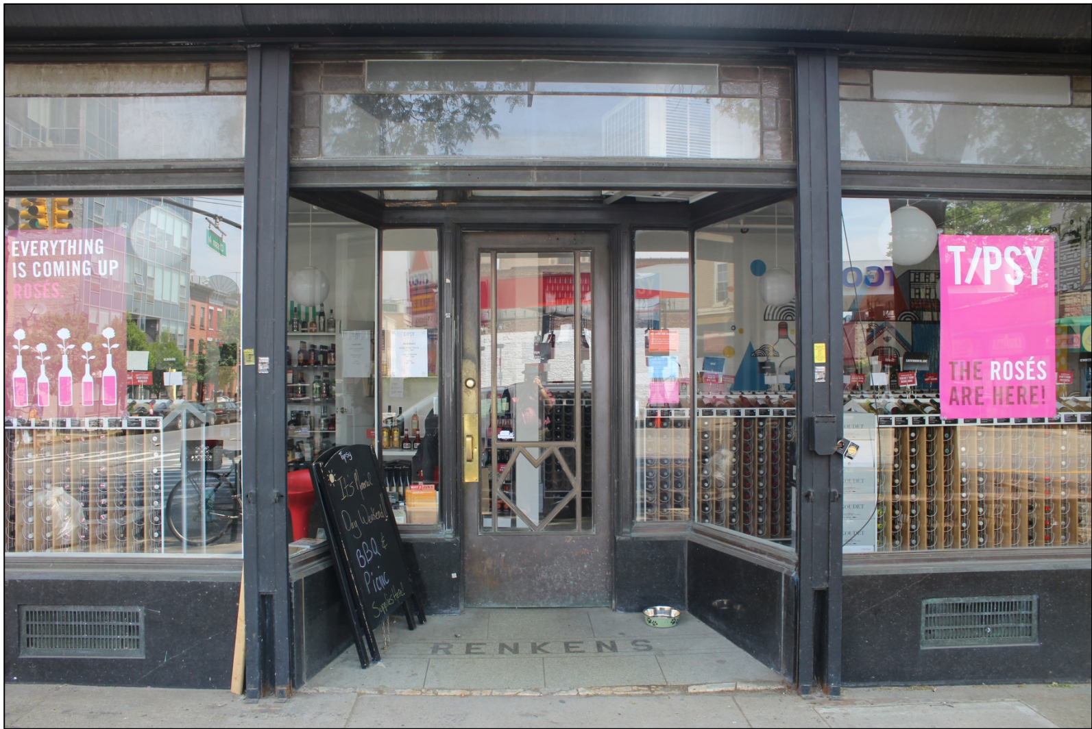
M.H. Renken Dairy Company Office Building Storefront
