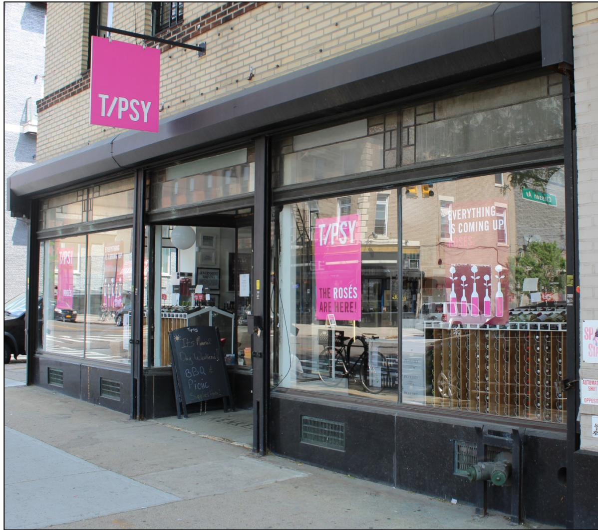
M.H. Renken Dairy Company Office Building Storefront
