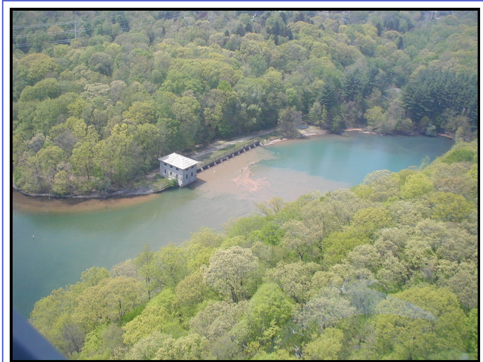
Figure 3.3 Photograph of the Catskill Influent Chamber Cove on Kensico Reservoir taken in May 2005 during alum treatment (looking approximately northwest).
