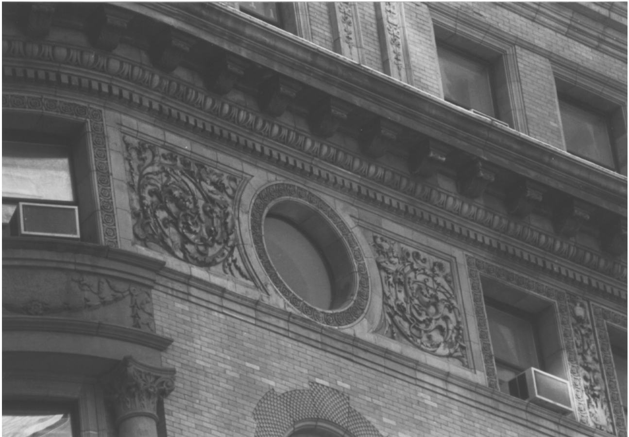
Delmonico's Building Details of the upper stories on Beaver Street Photos: Carl Forster
