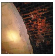
I snapped the photo above at one of the two points where the brick-lined New Croton Aqueduct meets the cast-in-place concrete of the Raw Water Tunnel. Brick is no longer used to build water and sewer mains, but the construction quality of the 19th-century New Croton Aqueduct is so
