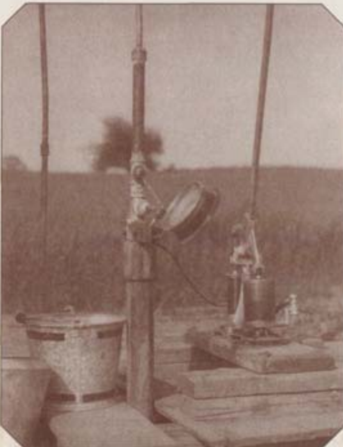
View showing details of testing apparatus at Walkill pressure tunnel. 1907
