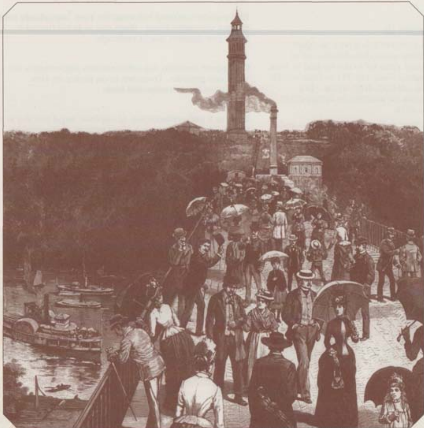
Croton Aqueduct High Bridge crossing over the Harlem River. View from the Bronx looking towards Manhattan where High Bridge Water Tower can be seen. Late 1800's
