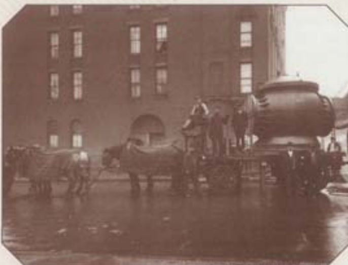
Bronze shaft cap, City Tunnel No. 1, Shaft 24, 1914
