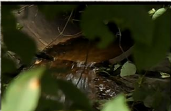
An outfall belonging to Yonkers near sentinel station S 61 discharging during dry weather.
