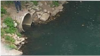
An outfall belonging to Yonkers at Nereid Avenue, discharging during dry weather.
