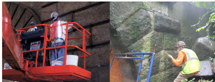
Pointing Joints on the East Face of the Brooklyn Anchorage of the Manhattan Bridge. Pointing the Masonry on the East Drive Bridge (East Wood Arch).
