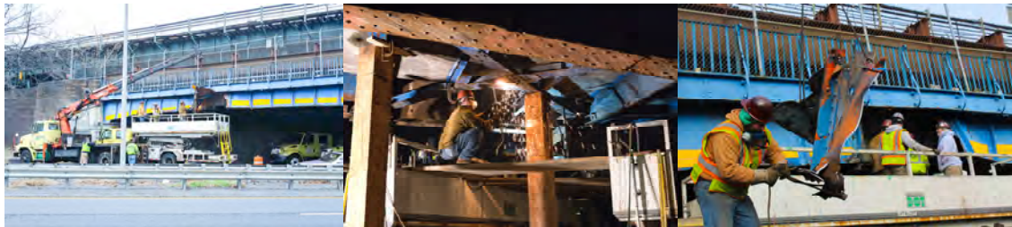
Damaged Bridge, Cargo Container, and Contractor Truck After An Over-Height Trailer Struck the Bridge in January 2012.
