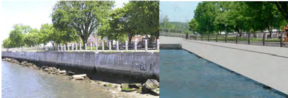
Existing Seawall. Proposed Treatment.
