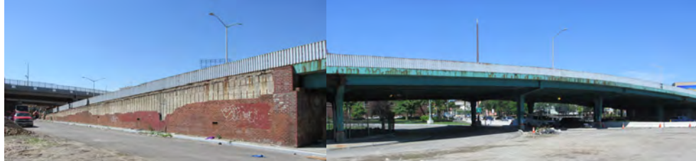
Project Location. 2014 - Left Elevation. 2015 – Right Elevation Spans 1-2 and 7-5. (Credit: NYSDOT)
