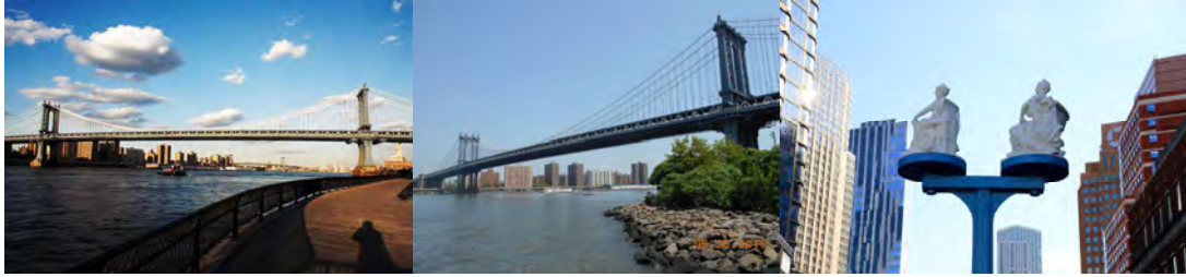
Manhattan Bridge in 2014 and 2016. (Credit: NYSDOT) Brain Tolle Designed Small Replicas of the "Miss Brooklyn" and "Miss Manhattan" Statues That Stood at Brooklyn Approach to the Manhattan Bridge Until the 1960's. The Statues Were Installed at the Flatbush Avenue Extension and Tillary Street in Late December 2016. The Resin Statues Rotate on Two Lamppost-Like Arms and are Illuminated From Within at Night. They are Set Back From the Entrance to the Bridge. This Project was Part of the Percent for Art Program. (Credit: Wendy Feuer)
