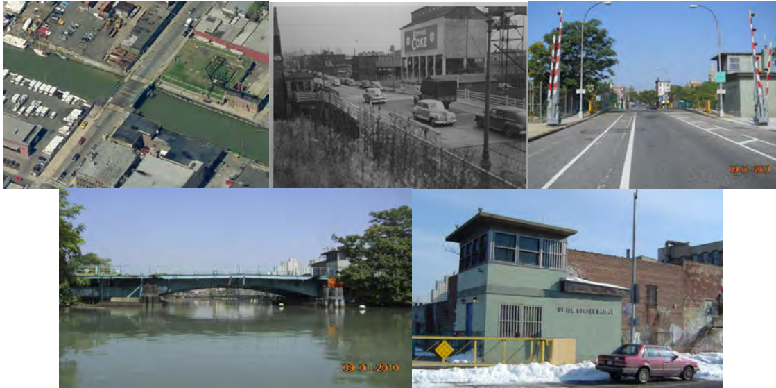
Aerial View of Union Street Bridge. Bridge in 1949 and 2010. (2010 Credit: NYSDOT) Operator House.
