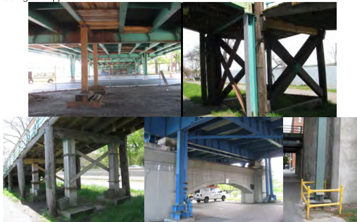
2014: Timber Shoring at Spans 7 and 8 of the Harlem River Drive over Ramp to and From Northbound Harlem River Drive. Steel Shoring of the Damaged Column at Pier 4 of the Crocheron Park Pedestrian Bridge. Timber Shoring at Piers 5 and 6. 2016: Steel Shoring at Span 5 of the East 174 th Street Bridge over the Sheridan Expressway. Eastbound Brooklyn-Queens Expressway over Washington Street – Shoring on the Right Side of the End Abutment.
