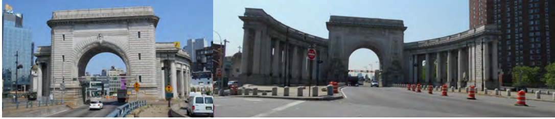
Manhattan Colonnade Begin and End Face in 2016. (Credit: NYSDOT)
