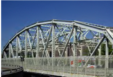
Macombs Dam Camelback Truss.
