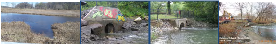
Turtle Cove. Existing Culvert – South Side.
