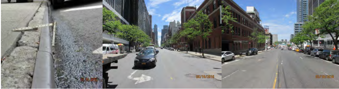
West 57 th Street Bridge over Amtrak. 2016: Beginning and Ending Approaches.
