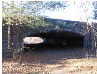
Mosholu Parkway Bridge over Equestrian Path. (Credit: NYSDOT)
