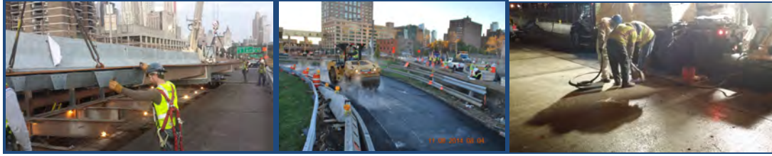
September 2014: Franklin Square Structure – New Orthotropic Deck. November 2014: Manhattan-Bound Brooklyn Approach Paving. December 2014: Super Slab Installation in Manhattan-Bound Lanes.
