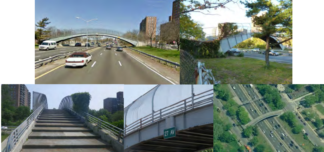
27 th Avenue Bridge – Existing Conditions.
