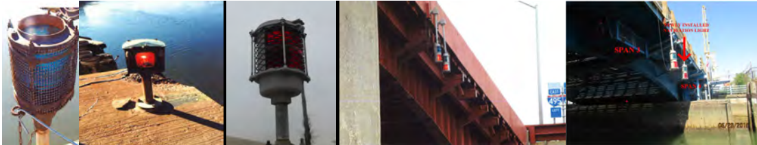
Northern Boulevard Bridge - Bridge and Pier Marine Navigational Lighting. Grand Street Bridge- Left Side Channel Light. Pulaski Bridge - Center Lights at Span #26. Third Street Bridge - Span #3. (Credit Grand and Third Street: NYSDOT)
