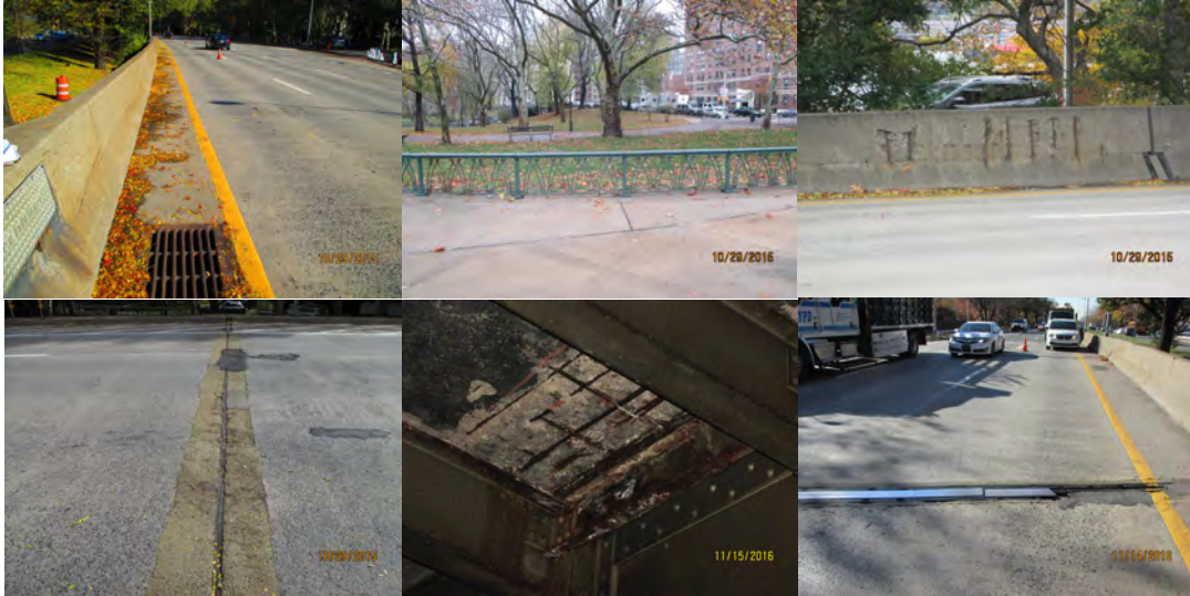
West 94 th Street Viaduct – 2015: Span 34 Left Lane. Span 12 Right Railing and Left Side Concrete Parapet. Span 31 Top of Deck. 2016: Span 4 – Spall With Exposed Rebar. Pier # 3, Deck Joint, Northbound Henry Hudson Parkway, Left Lane – Joint Missing Metal Plate. (Credit: NYSDOT)
