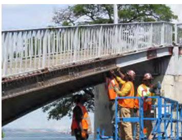
92 nd Street Pedestrian Bridge over Belt Parkway in August 2016 – Repairing Span #6.
