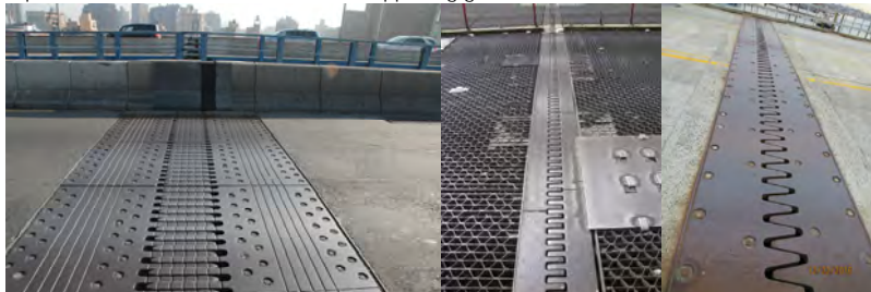
Manhattan Bridge Finger Dam. (Credit: Jagtar Khinda) Unionport Bridge Finger Dam at Span 9 in 2016. Riker's Island Finger Dam.
