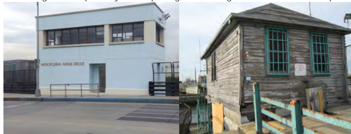
Metropolitan Avenue Bridge over English Kills and Grand Street Bridge Operator Houses. (Metropolitan Avenue Credit: Sunil Desai)
