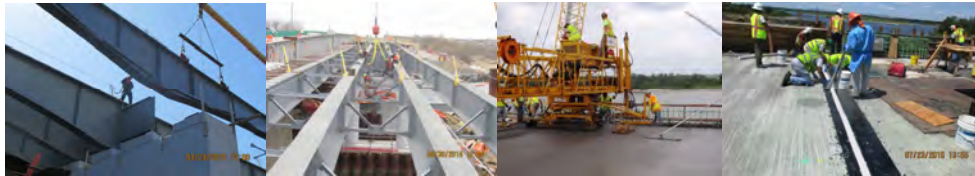
Gerritsen March 2015: Lowering a Girder onto the North Side of Pier #1 - Facing Southwest. April 2015: Four Girders With Diagonal Braces Set Between the East Abutment and Pier #2. June 2015: Placing and Finishing Deck Concrete. July 2015: Placing Armorless Joint in the Deck of the Westbound Bridge.
