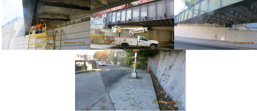
71 st Avenue Bridge Before, During, and After Construction.
