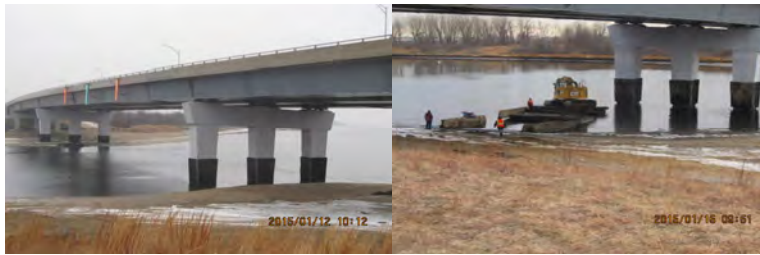
January 2015: Paerdegat Basin Bridges. Eastbound Belt Parkway Bridge over Paerdegat Basin. Newly installed Pier Bumpers at Low tide Facing East. Navigation Lights Over Center of Channel. Barge-Mounted Back Hoe used to Complete Installation of Pier Bumpers.
