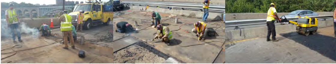
Repairing the Punch Through Holes on Top of the Deck.
