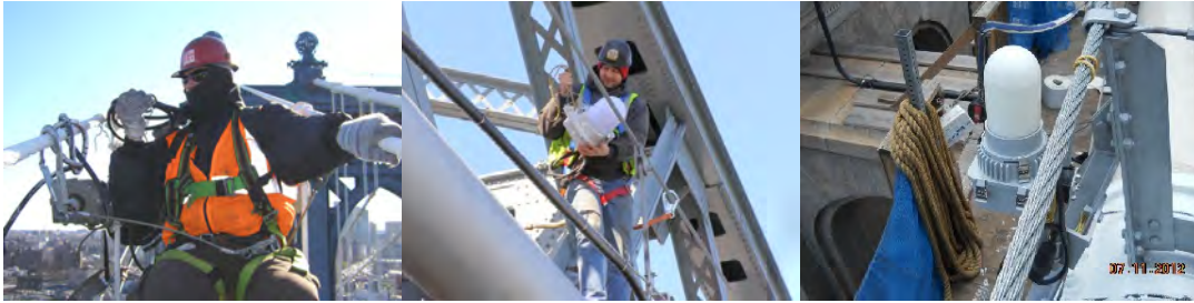
Repairing a Manhattan Bridge Necklace Light. Bridge Repairer and Riveter Neil Dalton Installing a New Light on the Williamsburg Bridge in 2012. (Credit: Hany Soliman) Manhattan Bridge Side Necklace Light. (Credit: NYSDOT)
