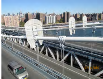
Suicide Gates on the Cables of the Manhattan Bridge. (Credit: NYSDOT)
