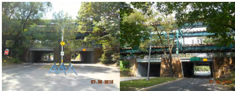
Roosevelt Avenue Bridge Over Flushing Meadow Park Road. July 2015: Elevation Left and Right. (Credit: NYSDOT)
