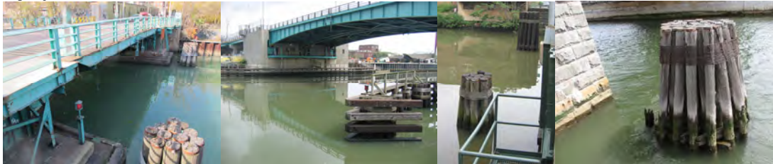
2014: Union Street Bridge Dolphins. Greenpoint Avenue Bridge Dolphin & Fender System. (Greenpoint Credit: Peter Basich) Hunters Point Avenue Bridge Dolphins. (Credit: Michele N. Vulcan) 145 th Street Bridge Dolphin. (Credit: NYSDOT)
