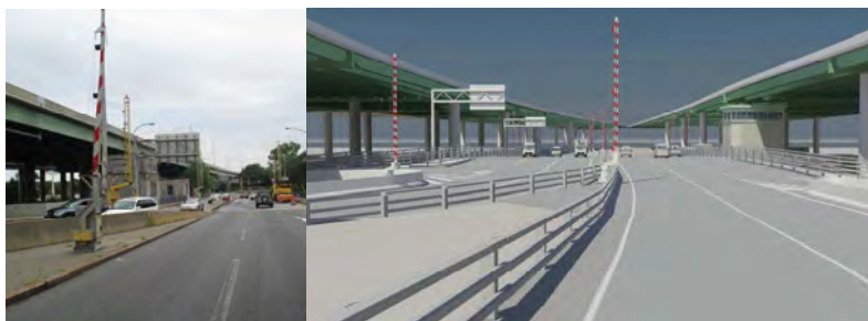
Looking East – Towards Current And Proposed Bridge.
