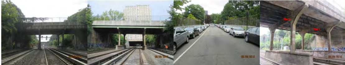
80 th Road Bridge over LIRR Main Line. September 2015: Elevation Left and Right. Begin Approach. Piers 1 and 2. (Credit: NYSDOT)
