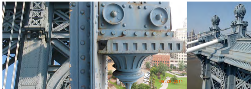
Ornamental Brackets, Rosette, Ball, and Cable Band.
