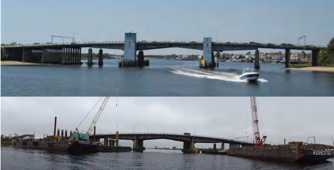
Mill Basin Bridge in 2010. (Credit: NYSDOT) Construction Site in October 2016.
