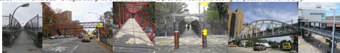
West 181 st Street, PS-5, Carroll Street over Franklin Shuttle, Chambers Street, and Staten Island Ferry (Over Parking Lot Exit Roadway) Pedestrian Bridges.
