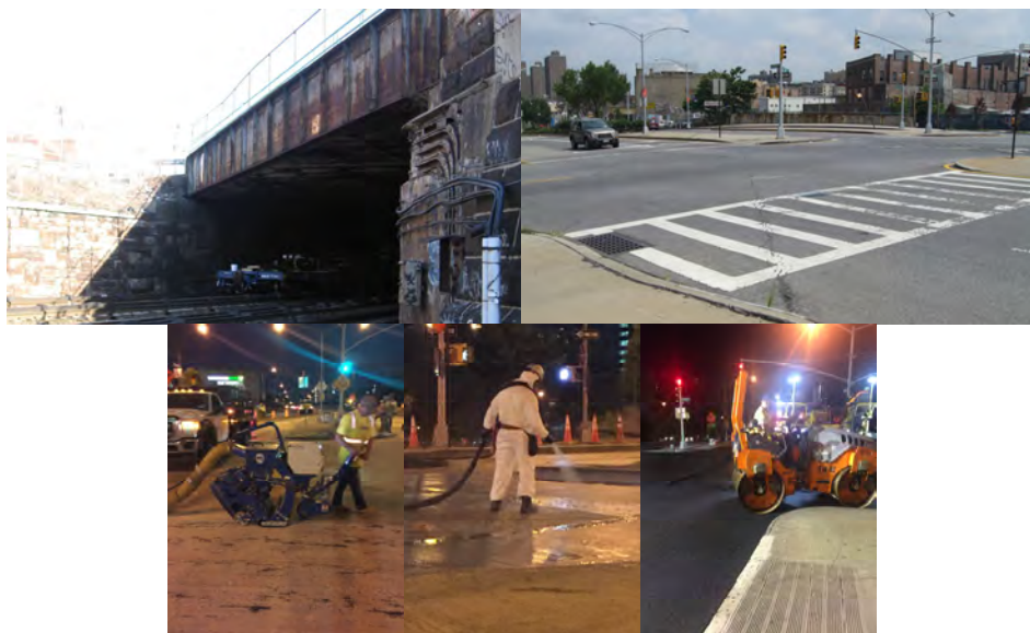
East 165 th Street Bridge over MNRR. July and August 2016.
