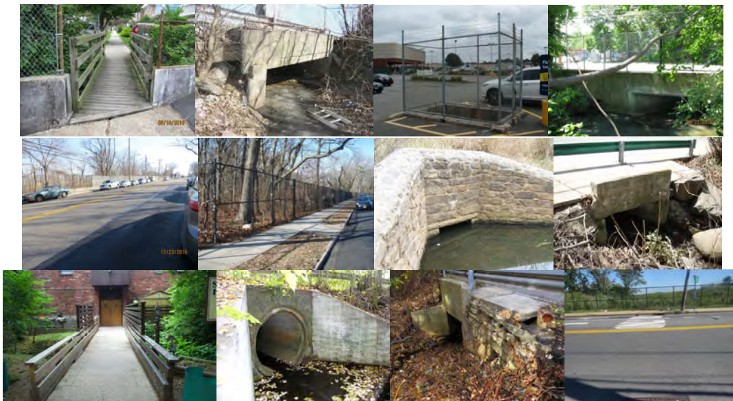
Galloway Avenue over Marianne Street – Wearing Surface, Looking Northwest. Forest Avenue over Crystal Avenue (2 Views). Midland Avenue over Hylan Boulevard (3 Views) – New Asphalt Wearing Surface. Culvert Top – Fence and Sidewalk. Rockland Avenue over Brielle Avenue. Forest Avenue over Randall Avenue. Gregg Place over Randall Avenue. Arthur Kill Road over Muldoon Avenue (2 Views). Arthur Kill Road over Ridgewood Avenue.
