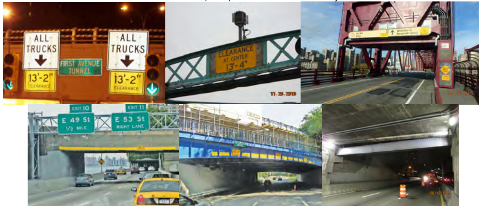
United Nations – 1 st Avenue Tunnel, Grand Street, and Roosevelt Island Bridge Vertical Clearance Posting. (Credit: NYSDOT) Retro-reflective Material Improves Visibility of These Low Vertical Clearance Bridges: East 60 th Street Bridge Over FDR Drive and Westchester Avenue Bridge over Hutchinson River Parkway. Vertical Clearance Beam at Span 53, Southbound Roadway of the Promenade over the FDR Drive. (FDR Credit: NYSDOT)
