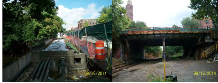
Ocean Avenue Bridge. September 2014. (Credit: NYSDOT)
