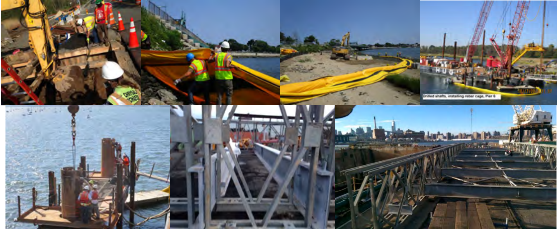
August 2014: Excavating on the West Side of the Bridge in the Presence of an Archeologist. Approximately 300 Linear Feet of a Turbidity Curtain was Installed on the Southwest Side of the Bridge to Protect the Shore During Construction. A Turbidity Curtain is a Floating Barrier Designed to Contain and Control the Dispersion of Sediment. October 2014: Drilled Shafts – Installing Rebar Cage at Pier 6. October 2014: The Contractor Airlifted Drilled Shaft Casings Into Position on a Platform Constructed Beside a Construction Barge. The Contractor Assembled the Temporary Bridge Segments at the Brooklyn Navy Yard. The Pieces Were Transported to City Island by Barge.
