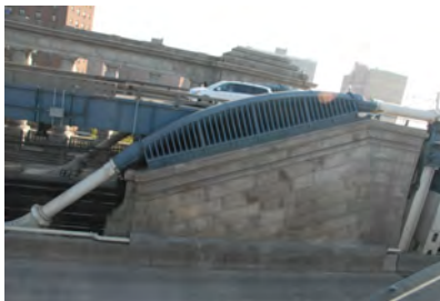
Manhattan Bridge Saddle. (Credit: Jagtar Khinda)
