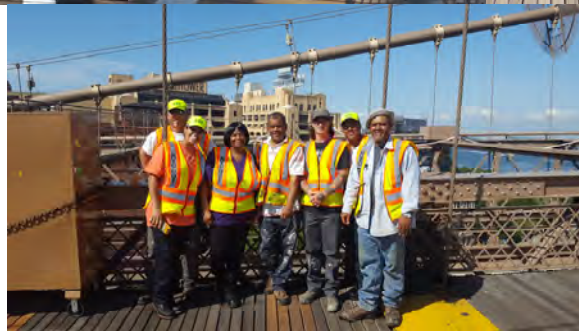
Brooklyn Bridge Line Striping in June and October 2016. (June Credit: Goncalo Lima) Bridge Painter Joice White. (Credit: Earlene Powell) July 2016: Bridge Painters John Gallagher and Joice White, Deputy Director of In-House Painting Earlene Powell, Bridge Painters Jamie Andrade, Sean Gabler, and Eduino Almada, and Supervisor Bridge Painter Goncalo Lima.
