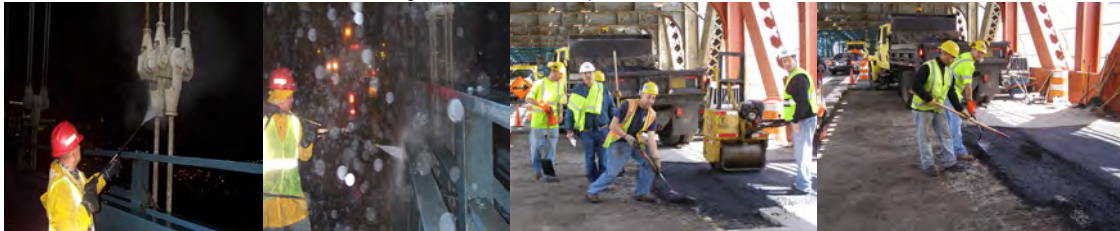
Power Washing the Corrosive Deicing Solvents Within the Range of the Roadway Splash Zone on The Manhattan Bridge in October 2007. Particular Attention is Directed to Cleaning the Gusset Plate. (Credit: Albert Hong) Performing Wear and Tear Resurfacing Work on the Roosevelt Avenue Bridges in April 2010: Assistant City Highway Repairer Victor Magagna, Supervisor Highway Repairer Joseph Palemine, Assistant City Highway Repairer Jonathan Adorno (Obscured), Assistant City Highway Repairer Anthony Montalbano, and Area Supervisor Highway Maintenance Edward Pedersen. Assistant City Highway Repairers Jonathan Adorno and Victor Magagna. (Credit: Joseph Flood)
