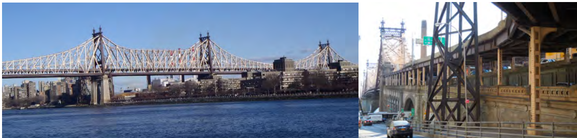
Ed Koch – Queensboro Bridge. (Credit: NYSDOT)
