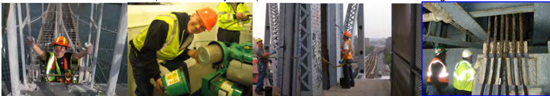
Assistant Mechanical Engineer Vera Ovetskaya Climbing to the Brooklyn Bridge Tower in 2008. (Credit: Gennadiy Kaplun) Oiler Tom Strommen Maintaining the Hydraulic Power Unit at the Hamilton Avenue Bridge in February 2010. (Credit: Vera Ovetskaya) Cleaning and Lubricating the Broadway Bridge. (Credit: Reza Taheri) Associate Project Manager Thomas Whitehouse (Wearing Yellow Jacket) Inspecting the Broadway Bridge Machinery Room and Instructing the Contractor. (Credit: Albert Hong)
