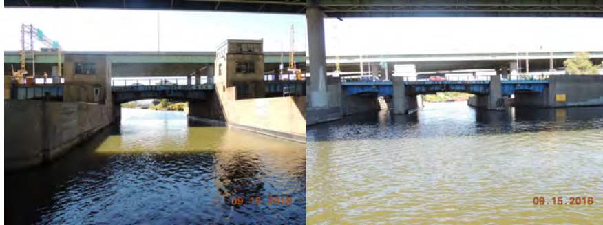
Existing Bridge in September 2016 – Left and Right Elevations. (Credit: NYSDOT)
