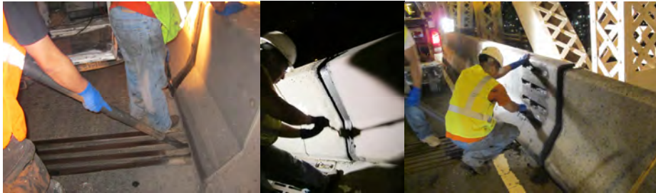
Expansion Joint Cleaning on the Williamsburg and Ed Koch - Queensboro Bridges in September 2011. (Credit: Shaikh Islam)
