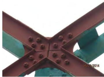
Grand Street Bridge Span 1 Truss Diagonal Member Gusset Plate.
