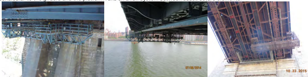
Manhattan Bridge and Ed Koch - Queensboro Bridge Travelers. (Credit: NYSDOT)
