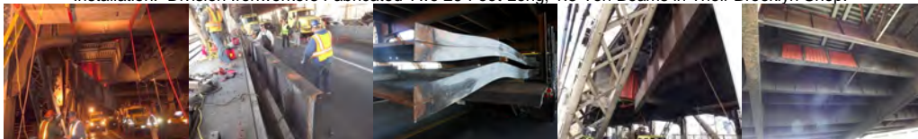
August 2013 Red Flags on the Ed Koch Queensboro Bridge. October 2013: Removing the Warped Beams. The New Beams.
