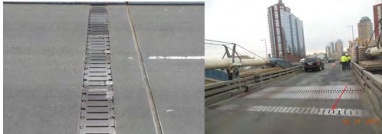
Manhattan Bridge Trench Drain.
