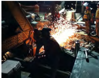
Welding Steel Packs for the Southbound Bruckner Expressway Bridge.
