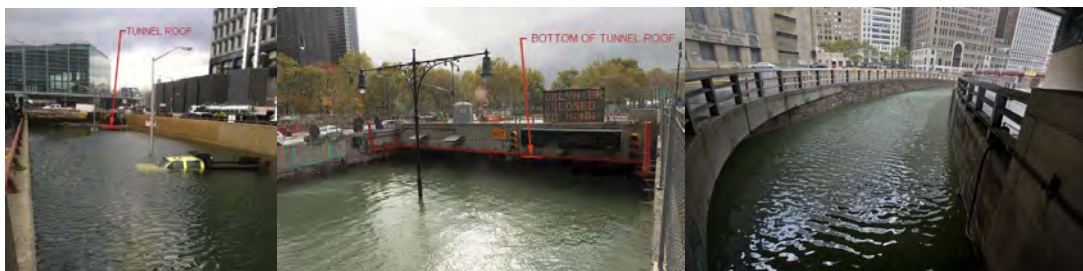
October 2012 - Battery Park Underpass - View Looking West at the South Portal Entrance Near the FDR Drive. View Looking South at the North Portal Entrance Near West Street. West Street Underpass – Approach at South Portal Looking Southeast. Both Tunnels Were Flooded to Their Roofs, Which Means That all Tunnel Ventilation, Electrical, and Mechanical Systems Were Entirely Submerged in Saltwater.
