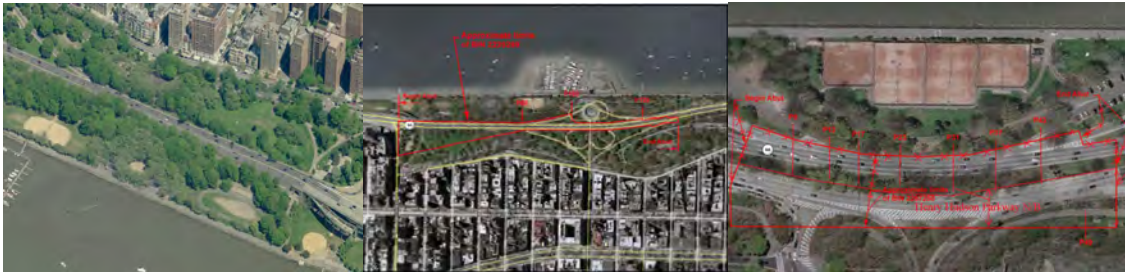
Aerial View of the Viaduct.
