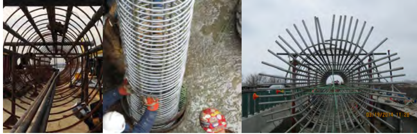
City Island, Gerittsen Inlet, and Bay Ridge Avenue Bridge Rebar Cages.
