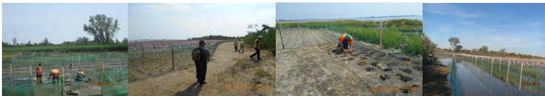
July 2013: Phase I Planting at the Bergen Beach Mitigation Area. August 2014: Grass Plantings Protected by Waterfowl Exclusion Fence. Placing the Plantings. Fence in October 2014.
