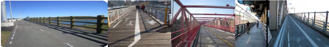
Fresh Creek Bicycle/Pedestrian Path in 2013. Brooklyn Bridge and Williamsburg Bridge Bicycle/Pedestrian Paths in 2010. (Williamsburg Credit: Russell Holcomb) Manhattan Bridge Bicycle Path in 2013. Ed Koch – Queensboro Bicycle/Pedestrian Path in 2016.
