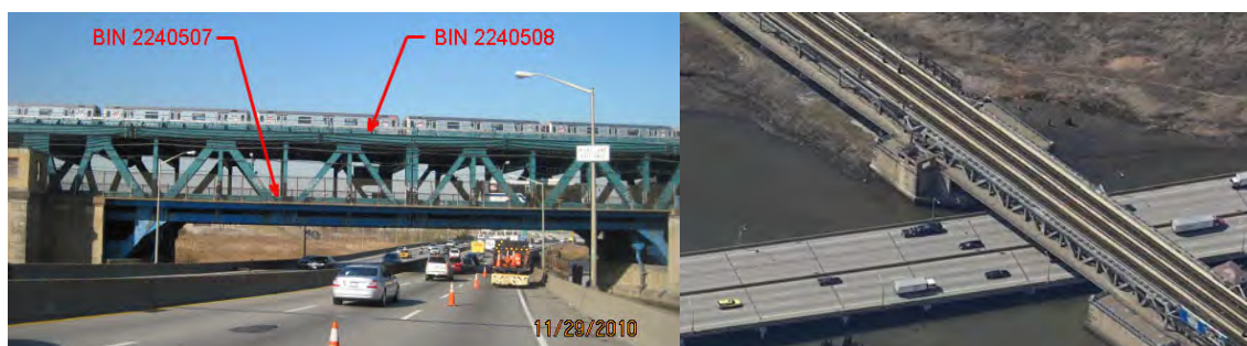
Roosevelt Avenue Bridge (#2240507) in 2010. (Credit: NYSDOT) Aerial View.
