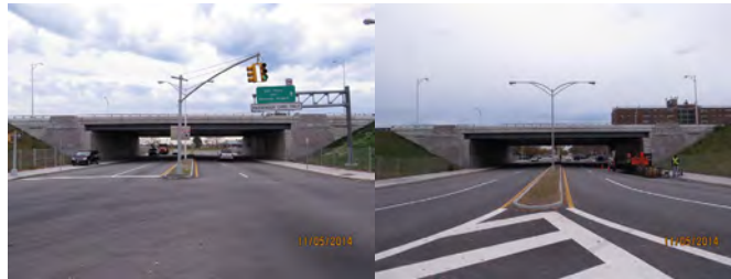
Rockaway Parkway Bridge in 2014: Left and Right Elevations. (Credit: NYSDOT)
