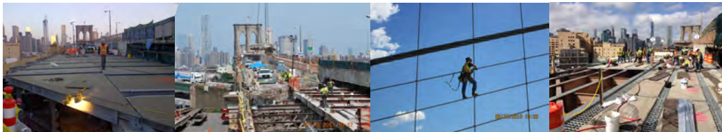
April 2013: Installation of Temporary Deck Units at the York Street Structure Over Brooklyn-Queens Expressway. July 2013: Removal of the Existing Concrete Slab on the Eastbound Main Street Structure. August 2013: Ironworker Replacing Cable Clamp Assemblies on the Suspended Span. October 2013: Grid Deck Panel Installation at the Eastbound Park Row Structure.
