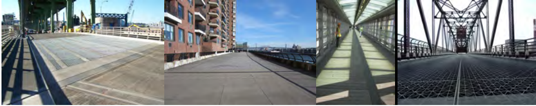
Hamilton Avenue Bridge, East 81 st to East 90 th Street Promenade over FDR Drive, Chambers Street Pedestrian, and Roosevelt Island Bridge Decks. (Hamilton and FDR Drive Credit: NYSDOT)
