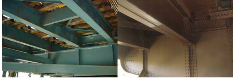
South Transit Floorbeams, Stringers, and Bracing Members on the Manhattan Bridge. Ed Koch Queensboro Bridge North Outer Roadway Floorbeam. (Credit: NYSDOT)
