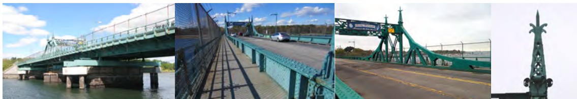
City Island Road Bridge in 2010. (Credit: Bojidar Yanev) Span 4, Right Sidewalk Near Pier 4 in October 2013. Vertical Clearance Posting. (Credit: NYSDOT) 9 Foot Tall Ornamental Finial.
