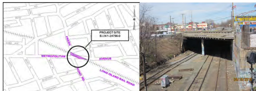
Location Map. Metropolitan Avenue Bridge in 2015.
