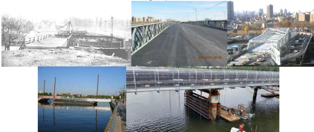
2011: Fresh Creek Temporary Bridge. 2004: Almost Completed New Third Avenue Span and Temporary Bridge. (Credit: Daniel Hom) 2005: Pontoon Bridge Used During the Emergency Reconstruction of the Ocean Avenue Pedestrian Bridge over Sheepshead Bay. (Credit: Russell Holcomb) 2015: City Island Temporary Bridge.
