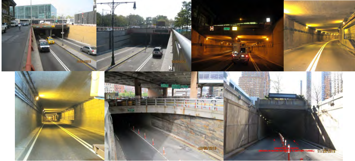
October 2013 – Battery Park Underpass – Elevation Right Span 1 and Left Span 1. (Credit: NYSDOT) September 2013 - Span 2 Looking Westbound (FDR Drive to West Street). June 2014 – The Underside of the Tunnel is Completely Covered With Tiles. October 2013 - West Street Underpass - Elevation Right Span. November 2015 – Left Fascia. (Credit: NYSDOT)
