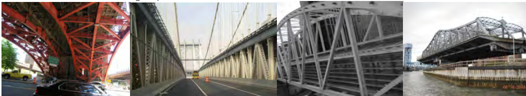
Brooklyn Bridge Franklin Square Truss. (Credit: Andy Hoang). General view of Manhattan Bridge Trusses B and C From the Lower Roadway on the Main Span. (Credit: NYSDOT) Chambers Street Pedestrian Bridge Truss. Madison Avenue Bridge Truss Swinging. (Credit: NYSDOT)
