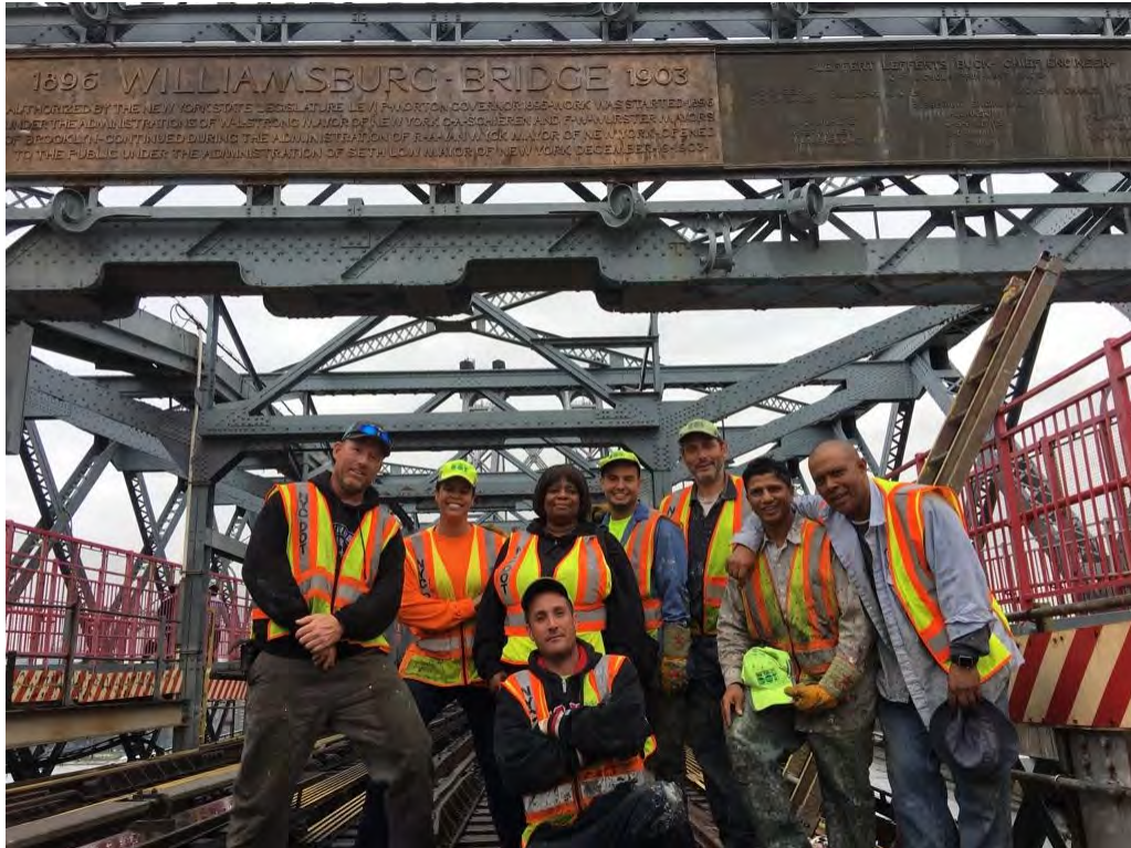
Bridge Painting Crew Pausing During the Removal of Graffiti From the Plaques on the Williamsburg Bridge in October 2016 – Bridge Painters John Gallagher and Joice White, Deputy Director of In-House Painting Earlene Powell, Bridge Painters Samuel Tejada and Konstantinos Issidoridis, Supervisor Bridge Painter Goncalo Lima, and Bridge Painter Steven Walsh in Front.. (Credit: Sammy Miraglia)
