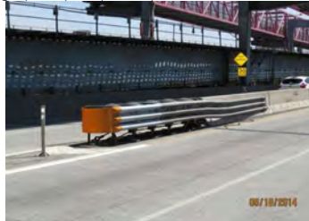
Williamsburg Bridge Impact Attenuator in 2014.
