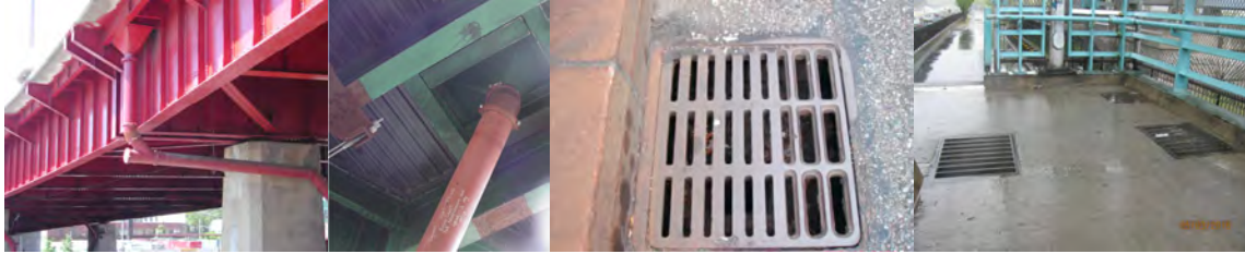
Scuppers on the Pulaski, Madison Avenue, and Brooklyn Bridges. (Credit: NYSDOT) Delancey Street Pedestrian Bridge – Span 8.
