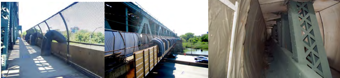
September 2016: - The Contractor Employs a Vacuum System to Capture Lead Particles During the Lead-Abatement Process. This is Done Using Negative Air Pressure to Prevent Emissions From the Abrasive Blasting Process Used to Remove Lead Paint. All Blasting is Done Within Negative Air Containment Units to Protect the Public From Emissions. View Inside the Containment – Bascule Span, Looking East.
