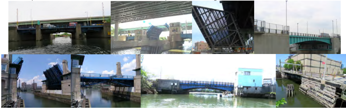
Unionport and Hamilton Avenue Bridge. (Open Credits: NYSDOT) Union Street Bridge. Greenpoint Avenue Bridge. (Greenpoint Credit: Michele N. Vulcan) Shore Road Bridge in July 2011. (Credit: Sergey Parayev) Metropolitan and Hunters Point Avenue Bridges.
