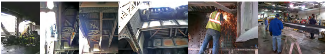
August 2013 Red Flags on the Ed Koch Queensboro Bridge. A truck caught fire on the bridge and damaged three stringers that support the eastbound upper roadway. Replacement of the two damaged stringers and the repair of a third were completed in October 2013. All work was performed by in-house forces. August 2013: Firefighters Examining the Damage. Repairing the Bridge Included Custom Designing the Steel Beams, as Well as Fabrication and Installation. Division Ironworkers Fabricated Two 26-Foot-Long, 1.5-Ton Beams in Their Brooklyn Shop.
