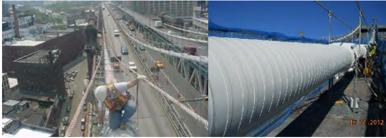
Inspector on Manhattan Bridge Cable. Cable B. (Credit: NYSDOT)
