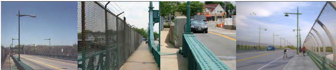
Existing and Proposed City Island Road Bridge Furnishings: Lighting, Fence, and Rail.
