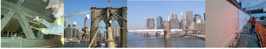
May 2013: Painter Applying Primer Stripe Coat on the Manhattan Main Span. June 2013: Painter on Sway Bracing on the Brooklyn Side Span. (View Credit: Earlene Powell) November 2013: Painting Fascia Steel on Ramp C.
