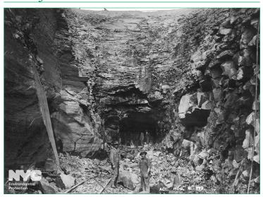
Looking into the south portal of the Catskill Aqueduct's Peak Tunnel on April 7, 1909, about a month after excavation began. All muck was removed by hand. Six months later, this heading met the one being excavated from the north portal about 3/4 of a mile away, making them the first tunnel headings to meet in the aqueduct.
