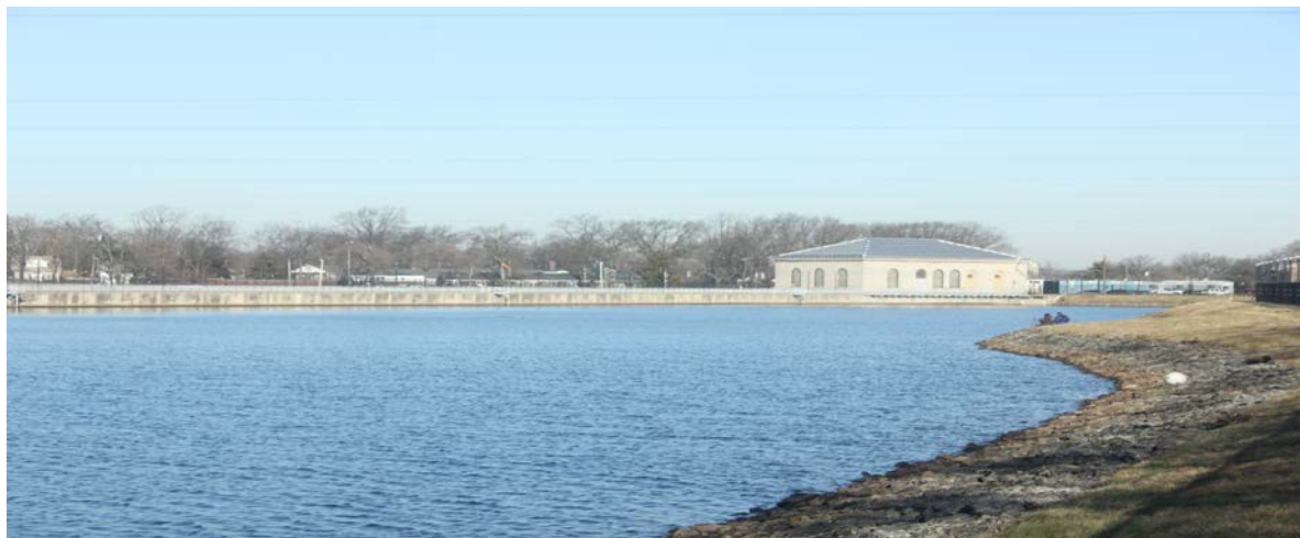
Figure 32. Hillview Reservoir overhead bird deterrent wires.
