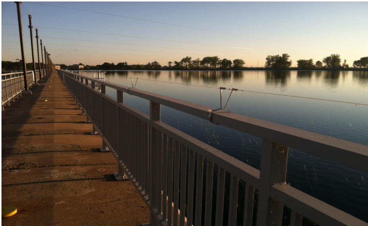
Figure 33. Hillview Reservoir bird deterrent wire system on dividing wall railing.
