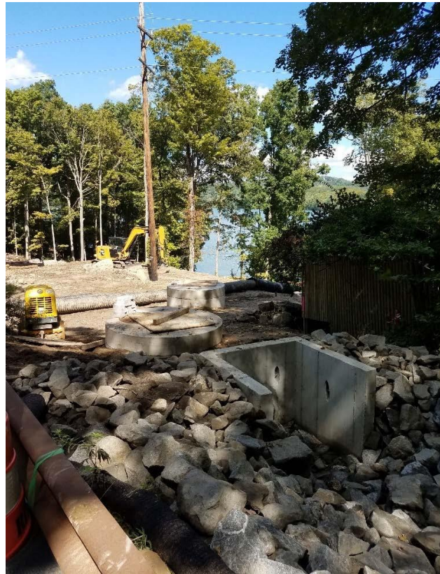
Figure 3.25 Site improvements at Maple Avenue retrofit.
