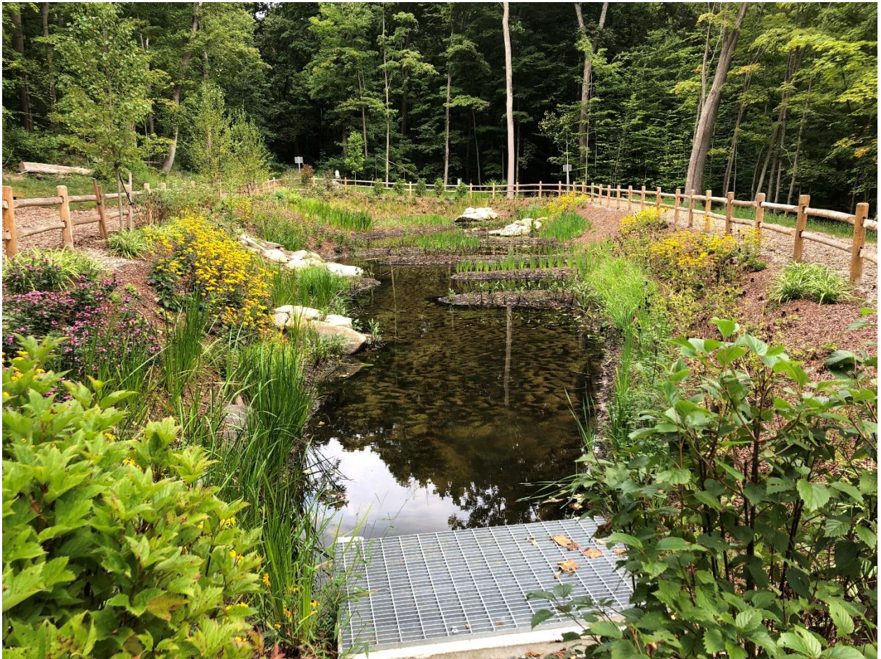
Figure 3.27 View of a pocket wetland in the Middle Branch Reservoir basin.
