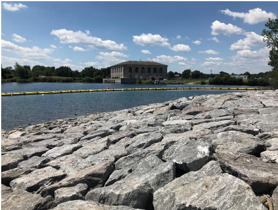
Figure 3.24 View of cove following placement of rip rap.
