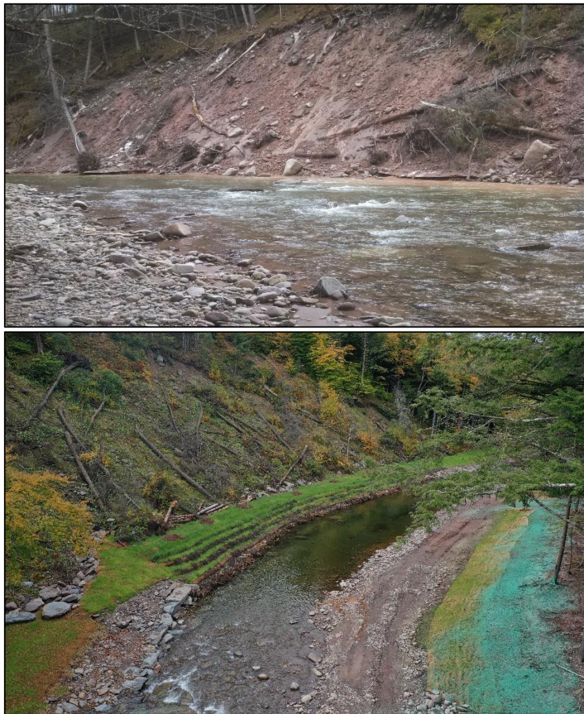
Figure 3.9 Clothes Pool project showing pre-construction conditions (top) and post-construction conditions (bottom).
