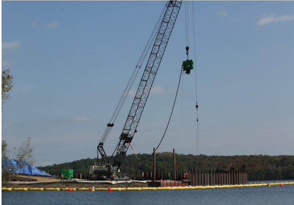
Figure 3.23 View of cove during installation of sheet piling.
