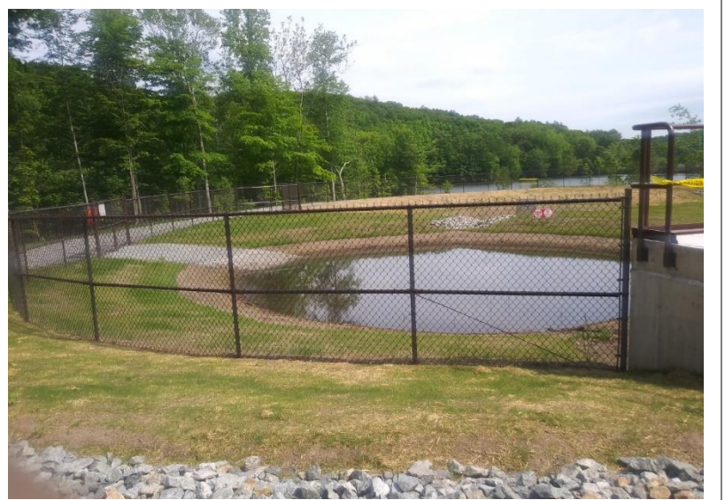
Figure 3.26 View of Drewville Road site
