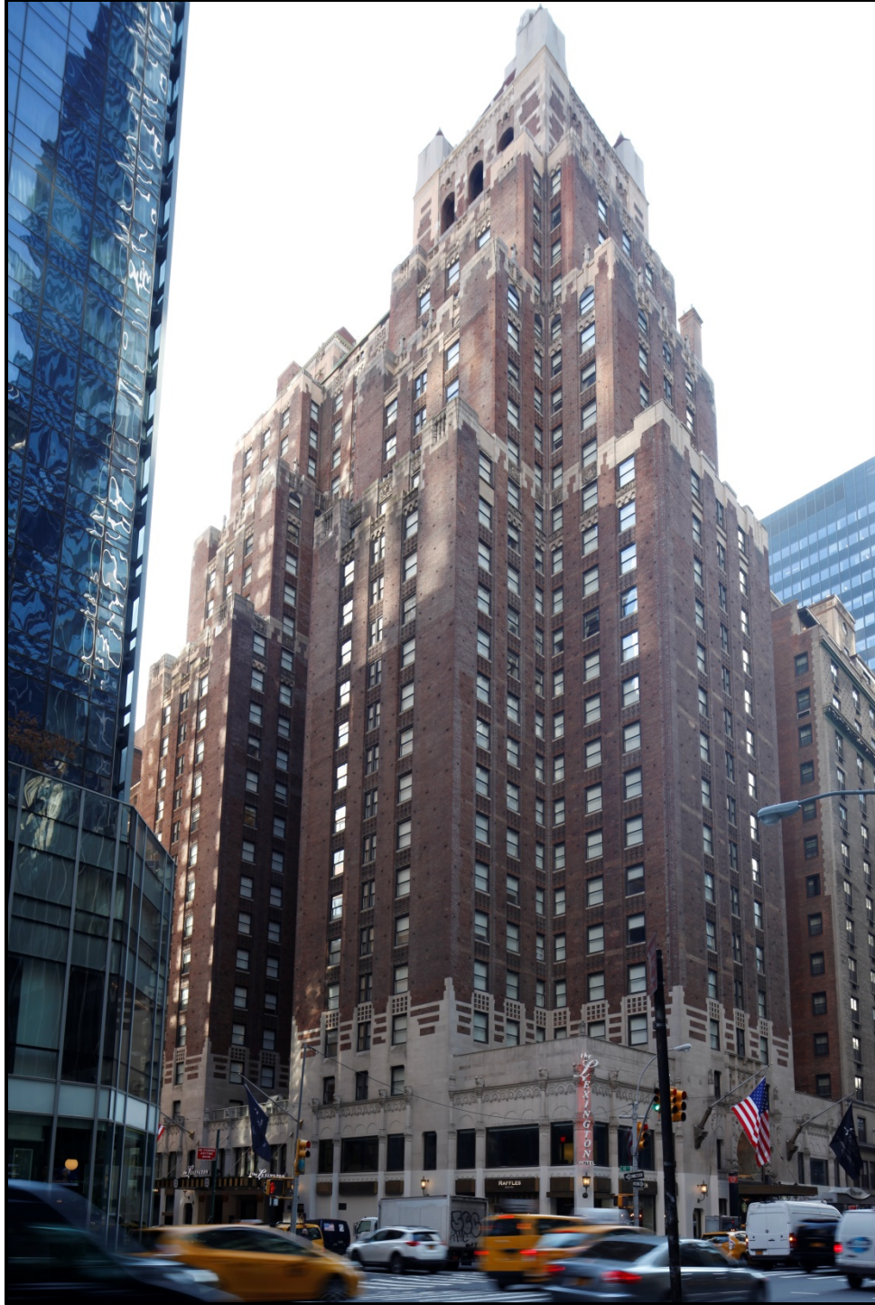
Hotel Lexington 511 Lexington Avenue (aka 509-515 Lexington Avenue; 134-142 East 48 th Street) Block 1302, Lot 51 Photo: Sarah Moses, 2016
