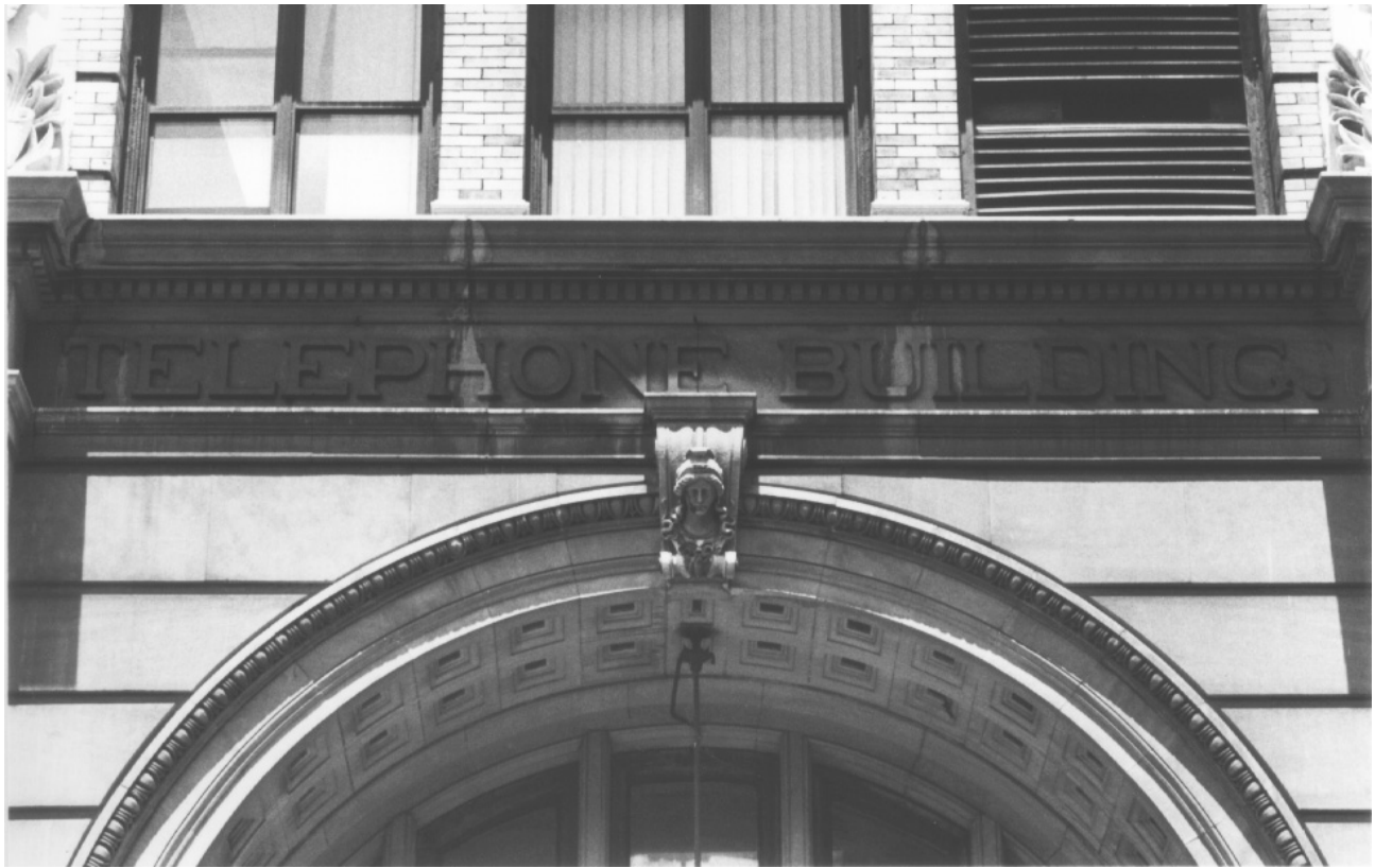
(Former) New York and New Jersey Telephone and Telegraph Building Ornamental details near entrance
