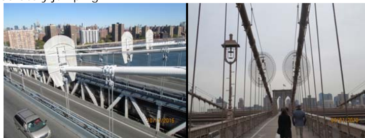
Suicide Gates on the Cables of the Manhattan (Credit: NYSDOT) and Brooklyn Bridges.
