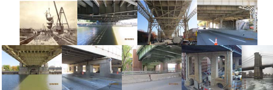
Madison Avenue Bridge Center Pier under Construction in September 1909, Pier 2 of Broadway Bridge. Piers 12, 33, 37, and 42 of Macombs Dam Bridge. (Credit: NYSDOT) Pier 1 (Looking East) of Hutchinson River Parkway Bridge over Hutchinson River. Pier 6 of Manhattan Bridge. Pier 39 of Brooklyn Bridge. (Manhattan and Brooklyn Bridge Credit: NYSDOT)
