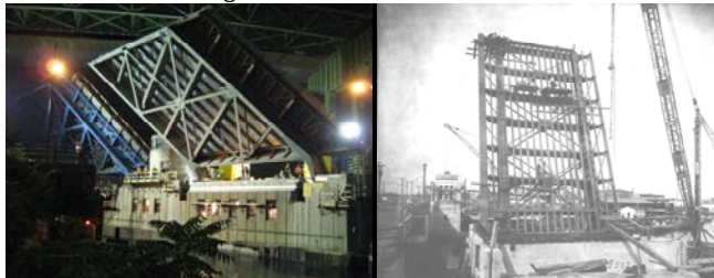
Leaves of the Hamilton Avenue Bridge. Cropsy Avenue Bridge Leaf under Construction in 1932.
