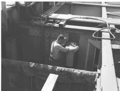
Engineer Using a Level on the Ed Koch - Queensboro Bridge in 1955.
