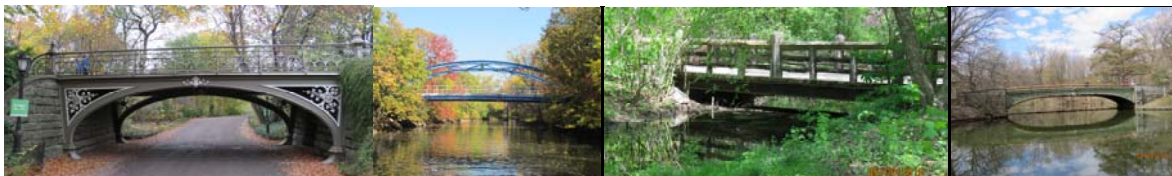
West 86 th Street Pedestrian Bridge (Southeast Reservoir Bridge) in 2018. Starlight Park Pedestrian Bridge over Bronx River in 2016. Music Grove Bridge and Lullwater Bridge in 2018 (in Prospect Park).
