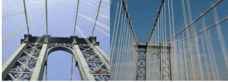
Manhattan Bridge Suspenders. (Credit: NYSDOT and Jagtar Khinda)
