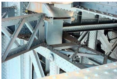
Truss Bearing on Manhattan Bridge. (Credit: NYSDOT)
