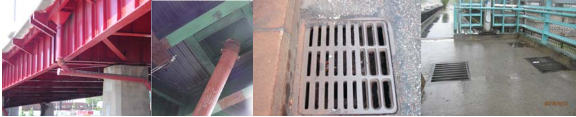
Scuppers on the Pulaski, Madison Avenue, and Brooklyn Bridges. (Credit: NYSDOT) Delancey Street Pedestrian Bridge – Span 8.
