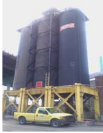
Hamilton Avenue Asphalt Plant Silo. (Credit: Sheena Diaz)
