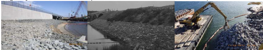
Riprap Installed in 2013 on South Side of Belt Parkway Bridge over Fresh Creek, Facing East. Riprap at the Southwest Side of the South Approach of the Shore Road Bridge over Hutchinson River in 1908. Barge-Mounted Crane Placing Riprap Stones on the South Slope of Gerritsen Inlet at the West Abutment in 2017.
