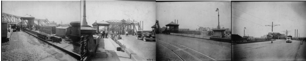
Constructing Guide Railing on the Madison Avenue Bridge in 1935.
