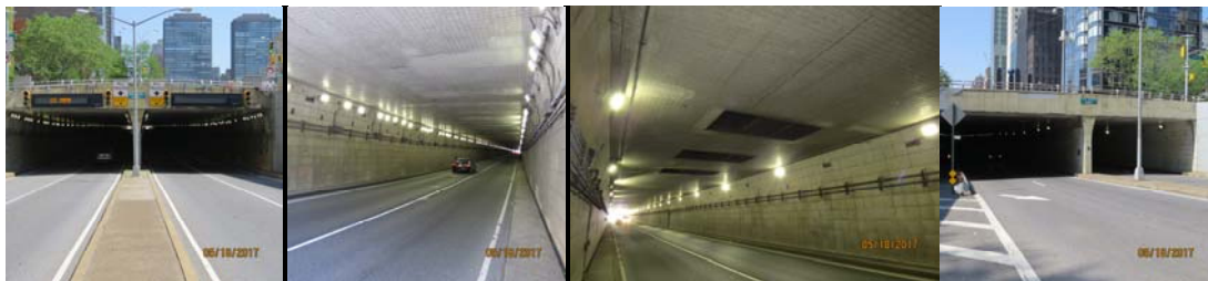
First Avenue Tunnel.
