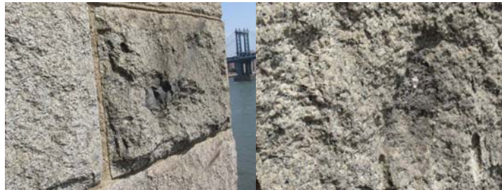
Brooklyn Bridge Tower Stone Scaling in 2016.
