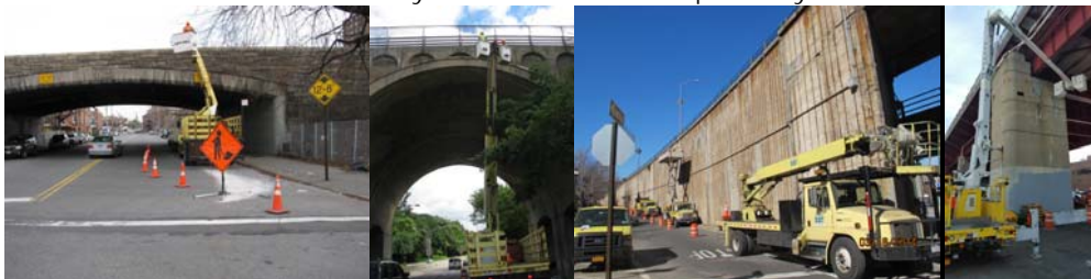
Inspecting the Belt Parkway Bridge over 26 th Avenue in December 2012. (Credit: Artemio Angeles) Nereid Avenue Bridge over Bronx River Parkway in June 2012 - Using a 60 Foot Boom with Outriggers. (Credit: Bojidar Yanev) Brooklyn-Queens Expressway (Eastbound) over Cadman Plaza/Brooklyn-Queens Expressway (Westbound). Pulaski Bridge in July 2017. (Credit: Mitul Patel)
