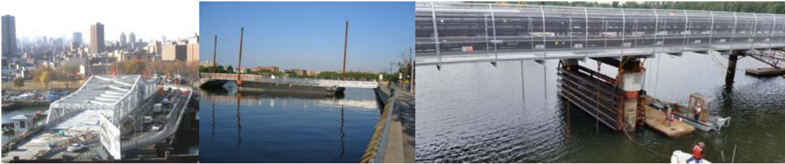
2004: Almost Completed New Third Avenue Span and Temporary Bridge. (Credit: Daniel Hom) 2005: Pontoon Bridge Used During the Emergency Reconstruction of the Ocean Avenue Pedestrian Bridge over Sheepshead Bay. (Credit: Russell Holcomb) 2015: City Island Temporary Bridge.
