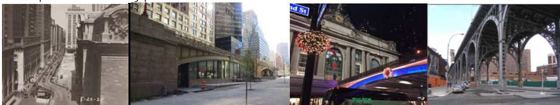
Park Avenue Viaduct Bridge – 1928 and 2018. (1928 Credit: NYC Records) Newly Installed Color-Changing LED Lighting in 2016. (LED Credit: MTA) Riverside Drive Viaduct.
