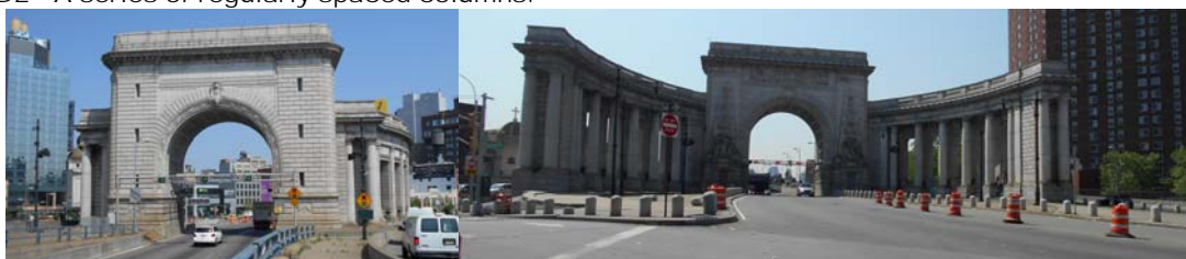
Manhattan Colonnade Begin and End Face in 2016. (Credit: NYSDOT)
