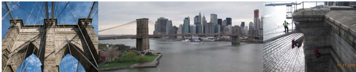
Brooklyn Bridge: 2009 Tower Closeup, 2010 View, 2010 Biennial Inspection. (2009 Credit: Emily Goodman, 2010 Credit: Jagtar Khinda, Inspection Credit: NYSDOT)
