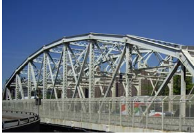
Macombs Dam Camelback Truss.
