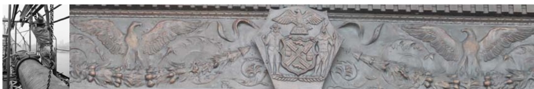
Manhattan Bridge - Replacing Cables in 1955. (Credit: NYC Records) Plaque Detail. (Credit: Peter Basich)
