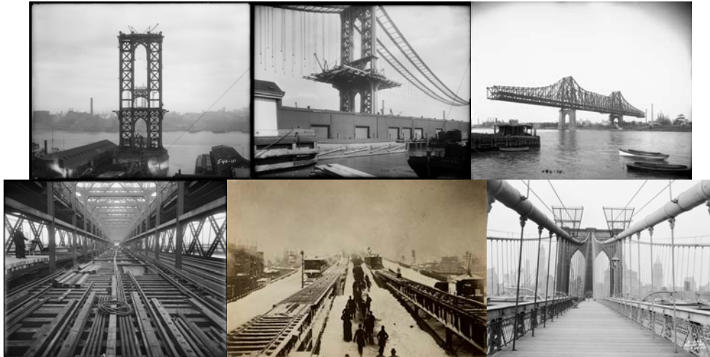
Manhattan Bridge under Construction in 1908 and 1909. Queensboro Bridge under Construction in 1920. Williamsburg Bridge in 1910. Brooklyn Bridge in 1888 and 1955. (Credit: NYC Records)
