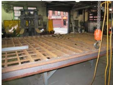
New Grizzly under Fabrication for the Agency Hamilton Asphalt Plant. (Credit: Russell Holcomb)
