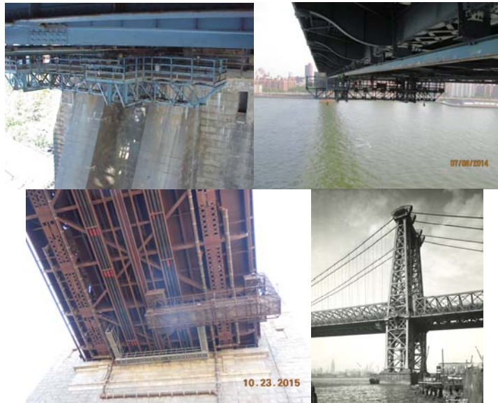
Manhattan Bridge and Ed Koch - Queensboro Bridge Travelers. (Credit: NYSDOT) Williamsburg Bridge in 1942: First Traveler in Place at the Brooklyn Tower. Second Traveler Shown on Scow Prior to Lifting.
