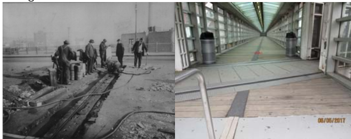
Constructing an Expansion Joint on the Riverside Drive Viaduct in 1918. Joint for Span 7 on the Chambers Street Pedestrian Bridge in 2017.
