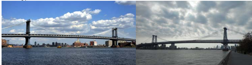
Manhattan Bridge. (Credit: Bernard Ente) Williamsburg Bridge in October 2016: Left Elevation Spans 24 – 28. (Credit: NYSDOT)
