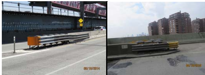
Williamsburg Bridge Impact Attenuators in 2014 and 2018.
