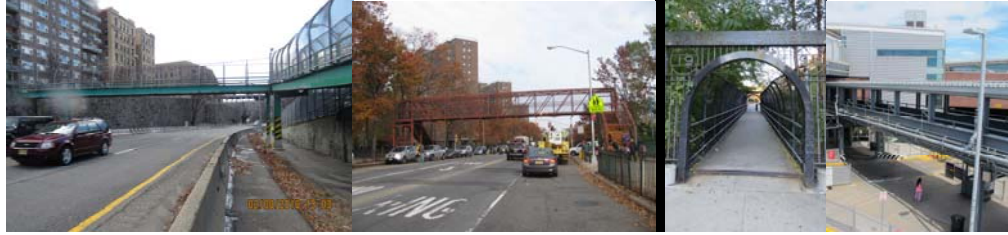
West 181 st Street, PS-5, Carroll Street over Franklin Shuttle, and Staten Island Ferry (Over Parking Lot Exit Roadway) Pedestrian Bridges.
