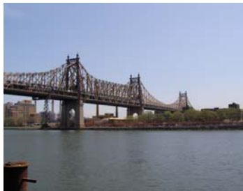
Ed Koch Queensboro Bridge. (Credit: Russell Holcomb)
