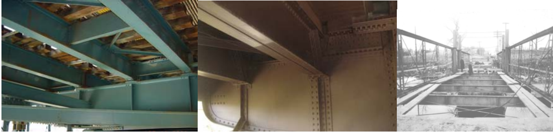
South Transit Floorbeams, Stringers, and Bracing Members on the Manhattan Bridge. Ed Koch Queensboro Bridge North Outer Roadway Floorbeam. (Credit: NYSDOT) Eastchester Bridge Floorbeams in 1914.
