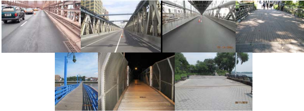
Brooklyn Bridge Wearing Surface. Manhattan Bridge Wearing Surface and Safety-Shaped Barriers. Williamsburg Bridge South Inner Roadway Wearing Surface. (Credit: NYSDOT) West 86 th Street Pedestrian Bridge (Southwest Reservoir Bridge) Wooden Wearing Surface. Ocean Avenue Pedestrian Bridge over Sheepshead Bay. 60 th Road Pedestrian Bridge over LIRR. Promenade over FDR Drive Span 43. (FDR Credit: NYSDOT)
