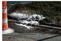
As the water was being pumped, Reinhartsen explained to the reporters that right now we need to fill the main so we're going to use a 6 inch bypass around the main valve and fill the main slowly to get all the air out. Russell stressed that you can't just put water in the main or the main will burst!
