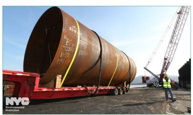
To eliminate leakage in a section of the Delaware Aqueduct, DEP is constructing a 2.5-mile bypass tunnel about 600 feet below the Hudson River, stretching from Newburgh to Wappinger. The new tunnel will be encased in 9,200 feet of steel. In early November, the first batch of massive steel liners arrived at a Hudson River port. In total, the project will require 230 sections of steel liner.
