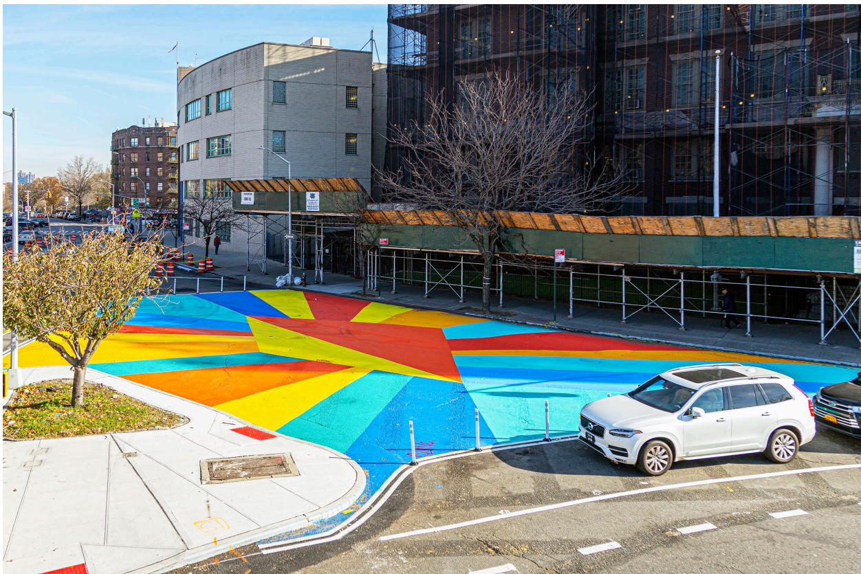
Macombs Road and University Ave, Bronx: Asphalt art mural at newly closed slip lane, new traffic signal, crosswalks, bus boarding island adjacent to Academy for Language and Technology, IS 232, IS 303, PS 204, and PS 723X
