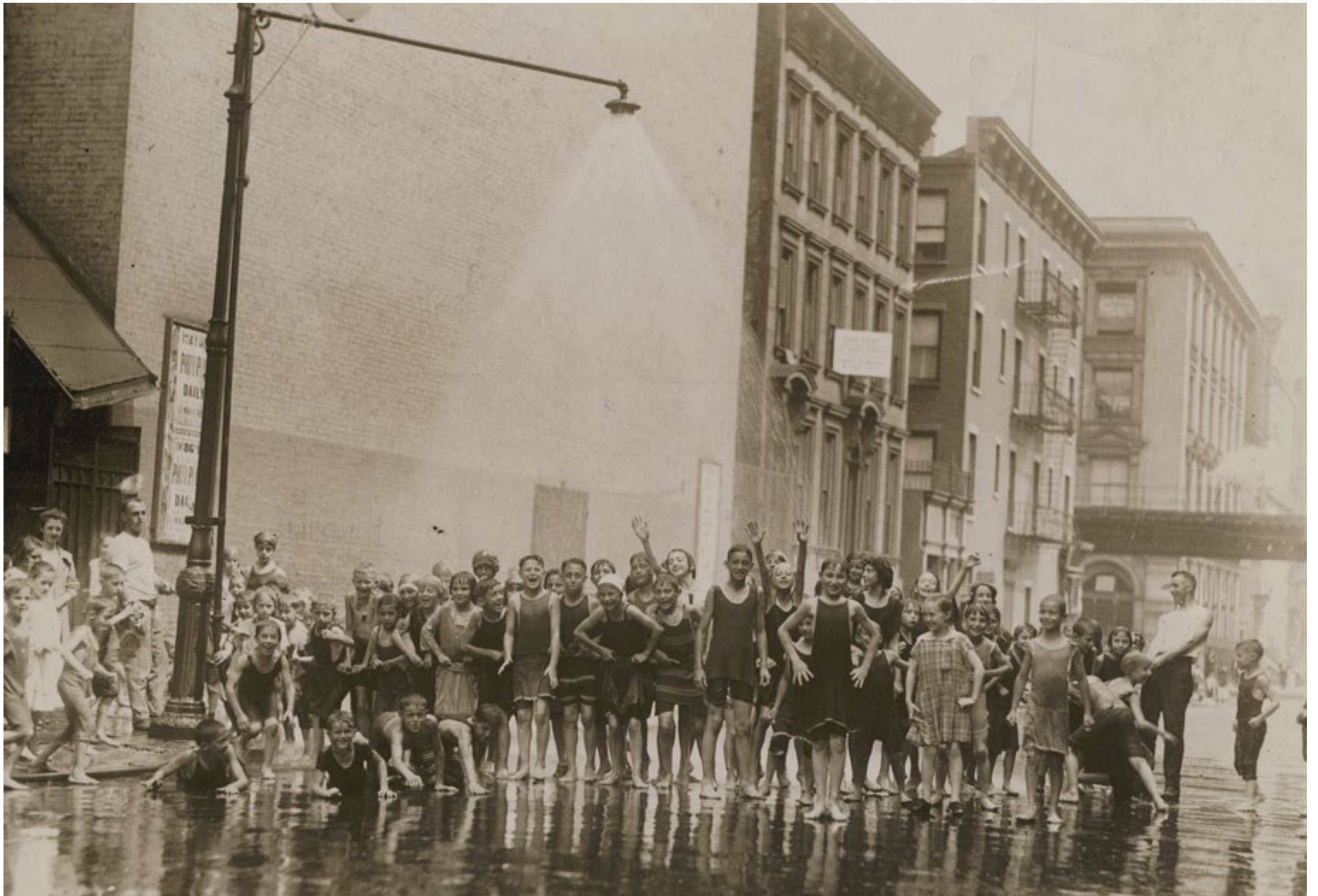
Mayors' Reception Committee Collection, FDNY Sprinkler, 85th St. near Lexington Avenue, August 17, 1920. Credit: International Newsreels/Film Service Inc.
