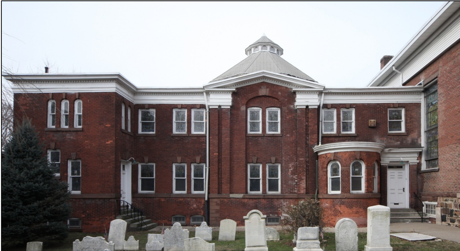
Reformed Church on Staten Island Sunday School Building Façade from east Photo: Christopher D. Brazee, 2010
