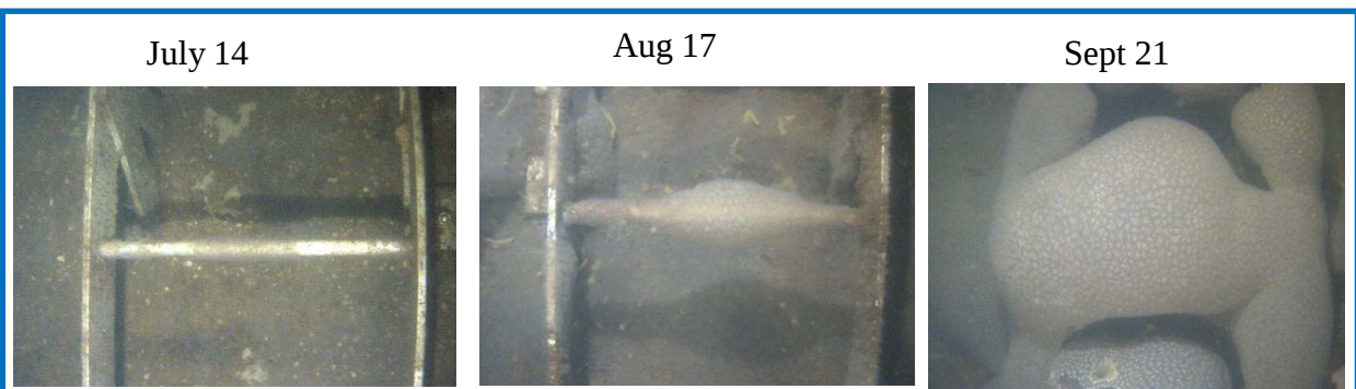
Figure 4.6 Photographs showing progression of P. magnifica colony growth on ladder rungs 12 and 13 at Delaware Shaft 18 in Sluice Gate 3 for 2014 to 2016. For scale, each of the ladder rungs are about 12 inches across.
