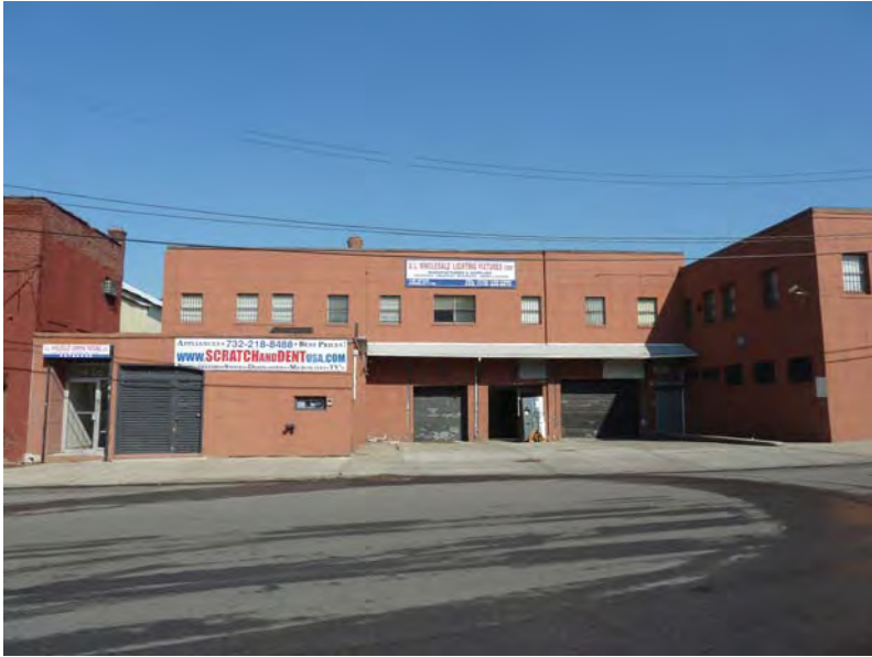
5. North view from 4th Street and 26th Avenue
