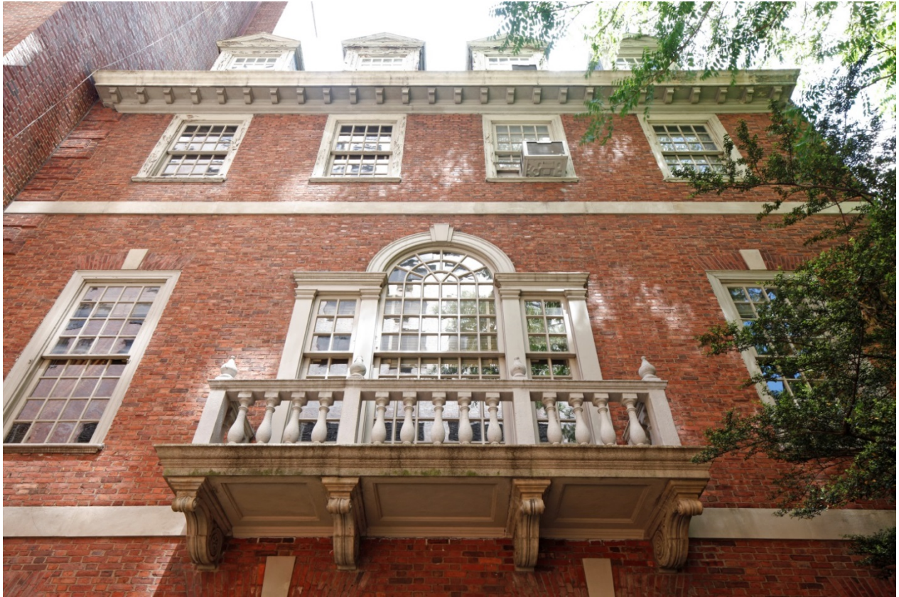
Rear facade, upper stories Sarah Moses, June 2019
