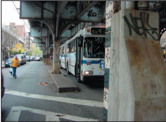
Alignment of columns and raised median at Westchester Avenue and Prospect Avenue
