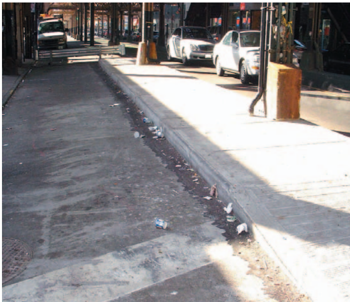
Raised median with guard rail protects pedestrians waiting for the bus
