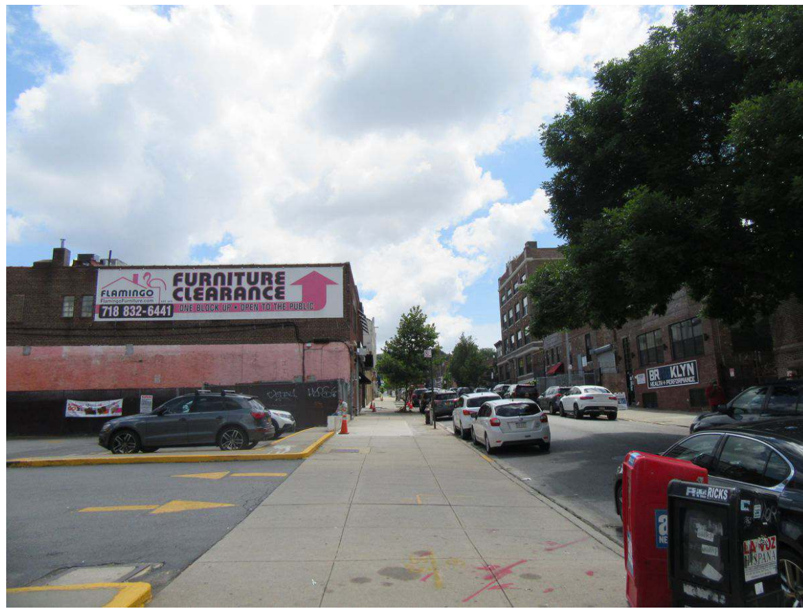
25. View of the sidewalk along the northeast side of 25th Street facing southeast from 4th Avenue (Development Site at left).
