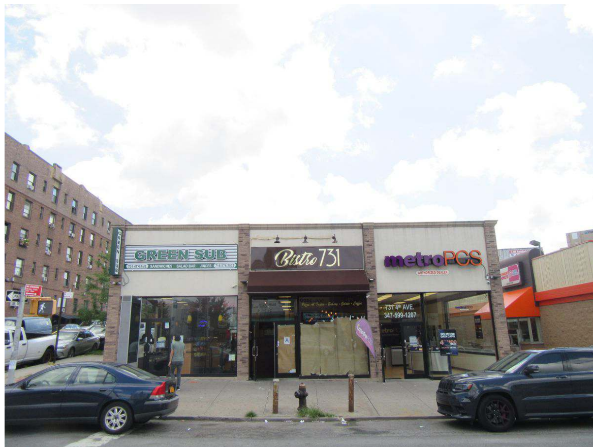
9. View of the Project Area facing southeast from 4th Avenue.
