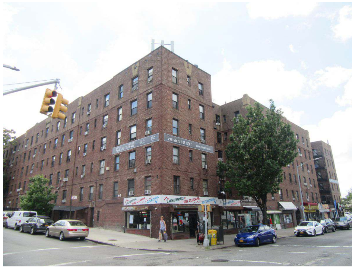
28. View of the intersection of 4th Avenue and 23rd Street facing south.
