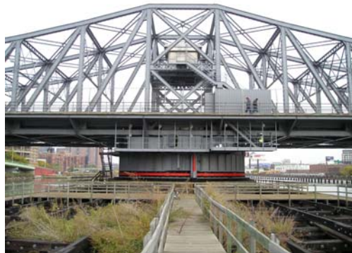
Freshly Painted Madison Avenue Bridge.
