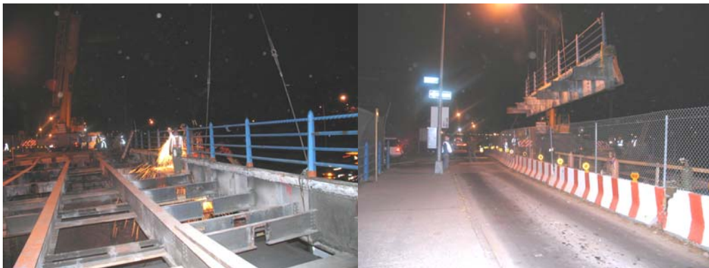
Structural Steel Removal on the Congress Street Bridge. (Credit: Carlos Ramirez)
