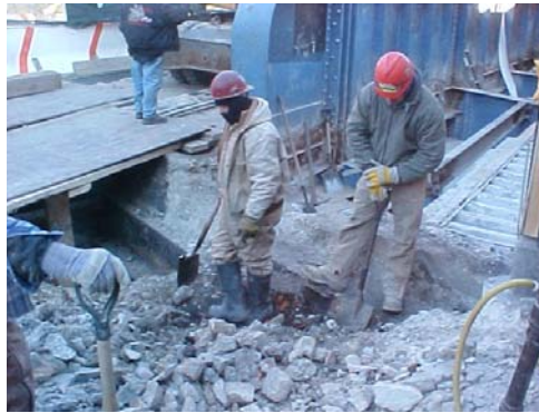
Excavating and Demolishing the Bridge Approach.
