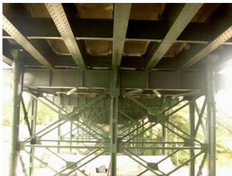
Detail of Freshly Painted East 241 st Street Bridge.
