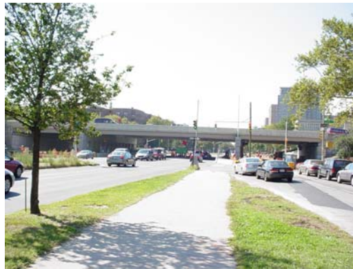
New Belt Parkway Bridge.
