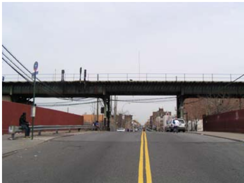
New Sutter Avenue Bridge.
