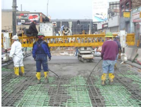
Deck Placement for the West 37 th Street Bridge.
