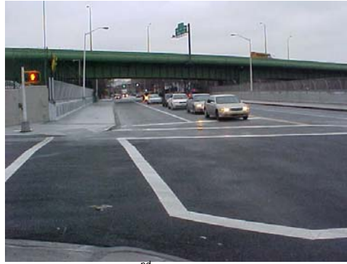
New 2 nd Avenue Bridge.
