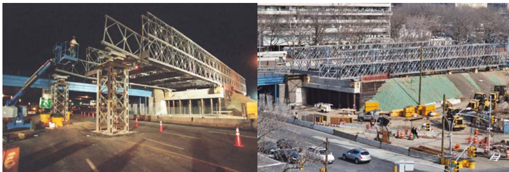
Temporary Belt Parkway Bridge.
