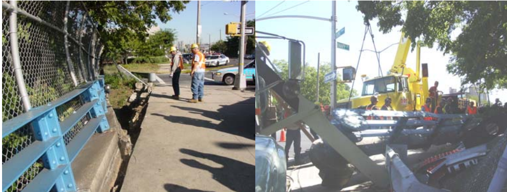
Division Personnel Inspecting the Damage. (Credit: Bala Nair)
