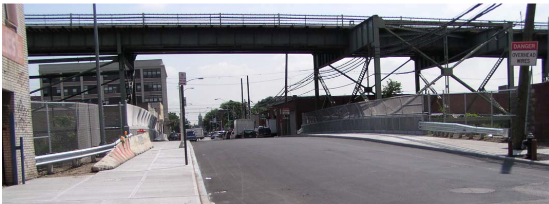
New Glenmore Avenue Bridge
