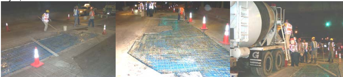
Division Crew Starting Concrete Deck Repairs. (Credit: Anthony Napolitano)
