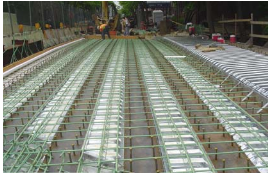
Installing Stay-in-Place Forms on the New Bridge.
