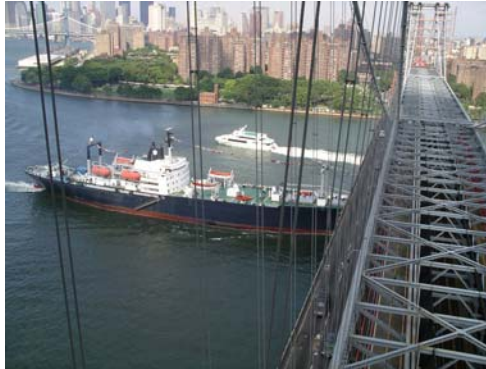
Looking East at the North Truss Top Chord.
