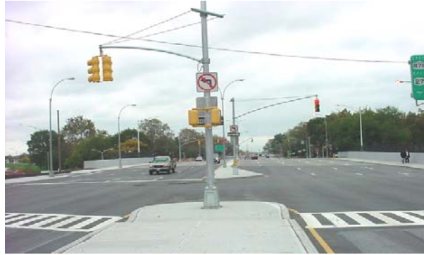
Looking South at the New Cross Bay Boulevard Bridge.
