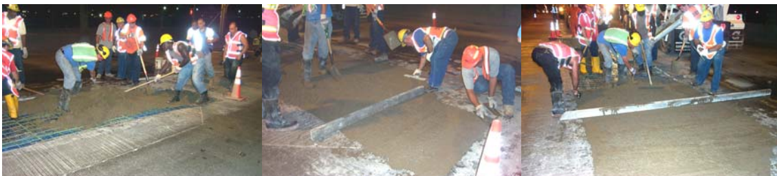
Division Crew Continuing Concrete Deck Repairs. (Credit: Anthony Napolitano)
