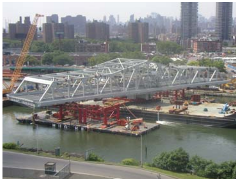
Transfer of the New Span From the Ocean to the Working Barges. (Credit: Daniel Hom)
