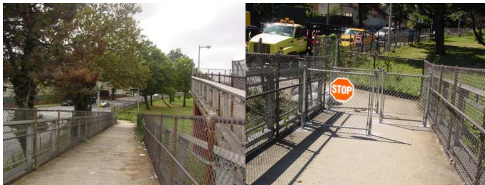
Bridge Ramp Before and After Installing the Fencing. (Credit: Hany Soliman)
