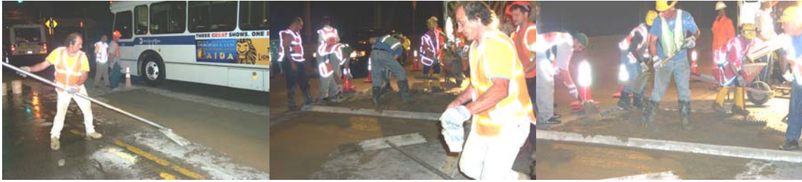
Division Crew Completing Concrete Deck Repairs. (Credit: Anthony Napolitano)
