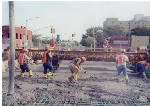
Placing the Deck Concrete.
