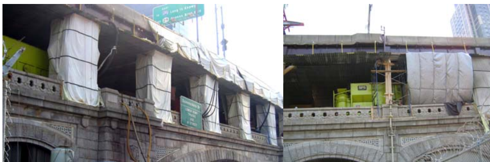
Containment on Queensboro Bridge Manhattan Ramp. (Credit: Peter Basich)
