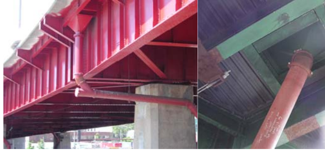
Scuppers on the Pulaski and Madison Avenue Bridges. (Credit: NYSDOT)
