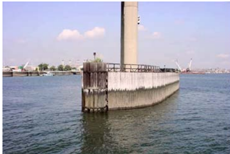
Rikers Island Dolphin & Fender System. (Credit: NYSDOT)
