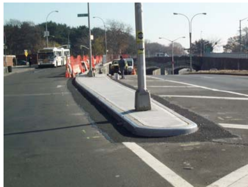
Repaired Bullnose Curb and Sidewalk at Crotona Avenue. (Credit: Joseph Saverino)
