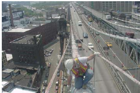
Inspector on Manhattan Bridge Cable. (Credit: NYSDOT)
