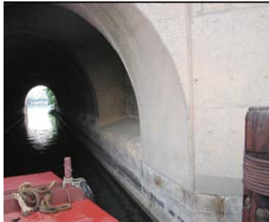
Hamilton Avenue Bridge Abutment. (Credit: NYSDOT)
