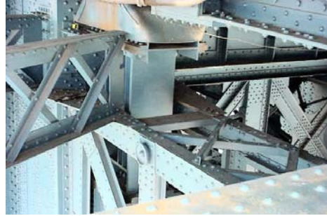
Truss Bearing on Manhattan Bridge. (Credit: NYSDOT)
