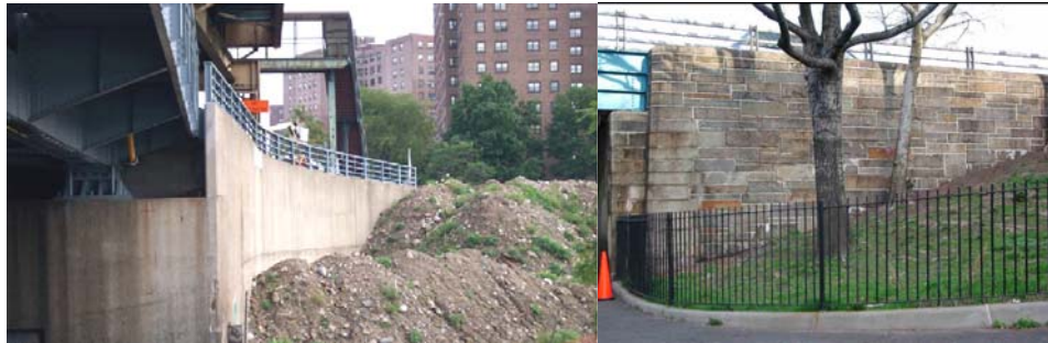
Broadway Bridge & Bay Ridge Avenue Bridge Wingwalls. (Credit: NYSDOT)
