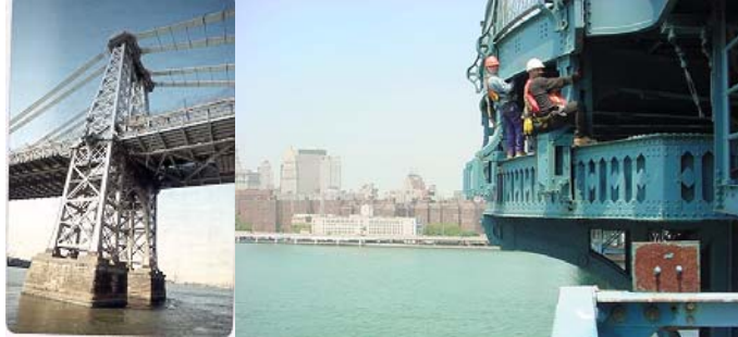
Williamsburg Bridge Tower. Inspectors on Manhattan Bridge Tower. (Manhattan Credit: NYSDOT)
