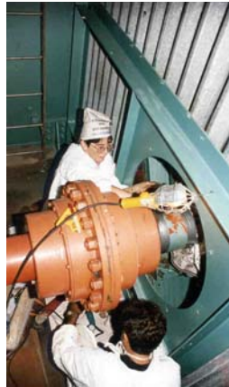
Division Engineers Installing Strain Gauges in 1995 on the Greenpoint Avenue Bridge
