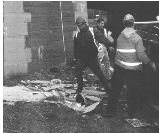
Hutchinson River Parkway Under Westchester Avenue. (Credit: Anthony Napolitano)
