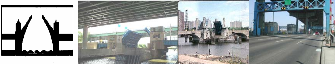
Unionport, Pelham, and Hamilton Avenue Bridges. (Unionport and Hamilton Credit: NYSDOT)
