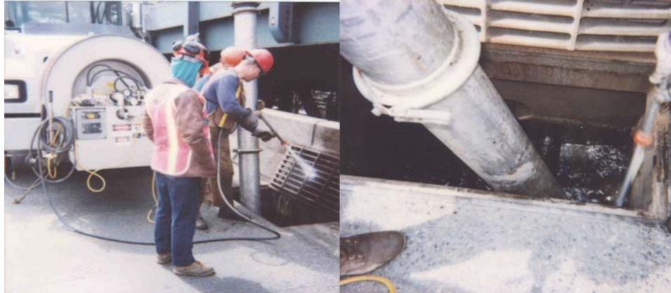
Cleaning Catch Basins on the Manhattan Bridge
