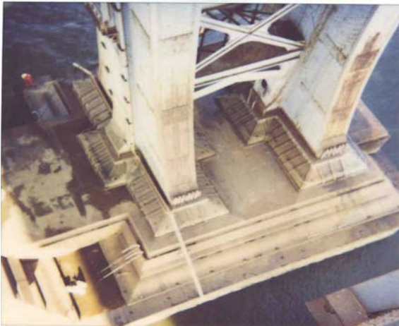
Manhattan Bridge Tower After Debris Removal
