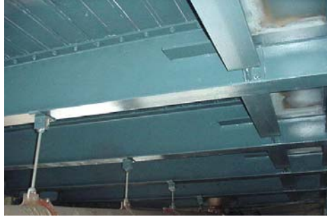
Stringers on the Manhattan Bridge. (Credit: NYSDOT)
